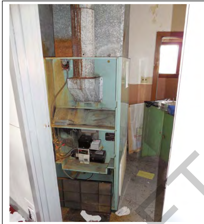
Photo 5: Oil-fired forced-air furnaces are located in each of the two storage rooms near the altar. (September 9, 2013)
