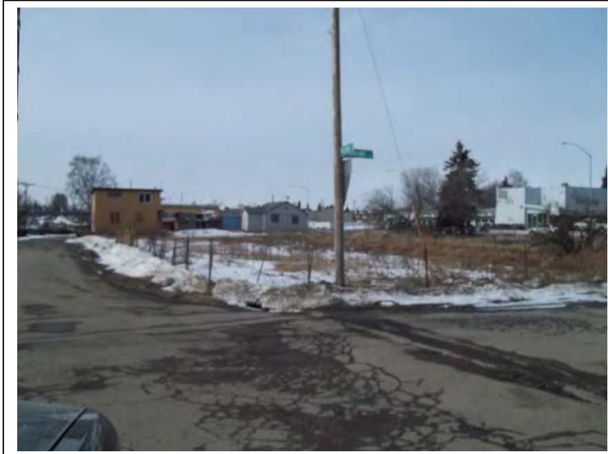
Photo 29: Deteriorated pavement; looking northeast. (April 18, 2014)
