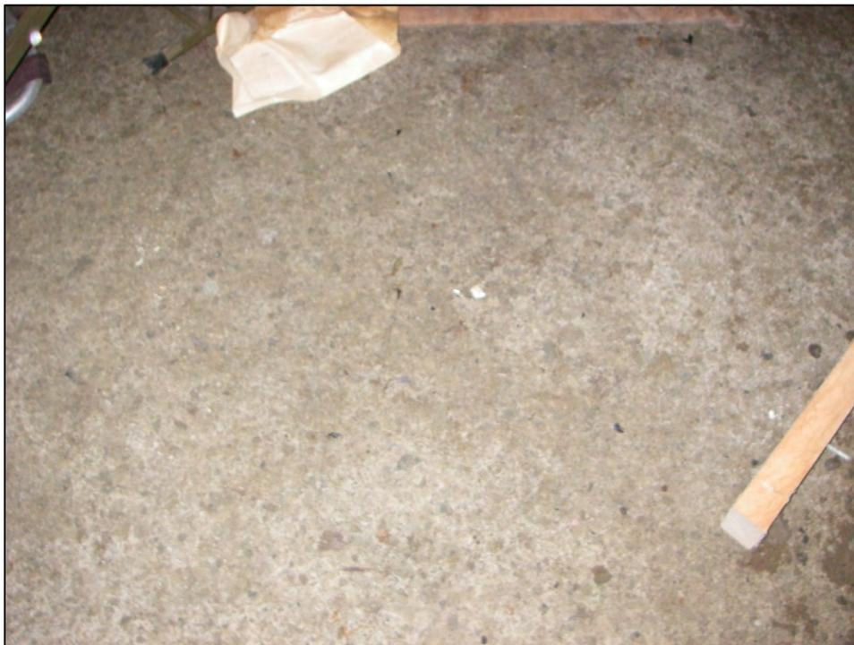
**PHOTOGRAPH 28: HARD-PACKED DIRT ON FIRST FLOOR OF OLD FIRE HALL BEHIND THE SAND PILE AND UNDER THE LOFT.**
