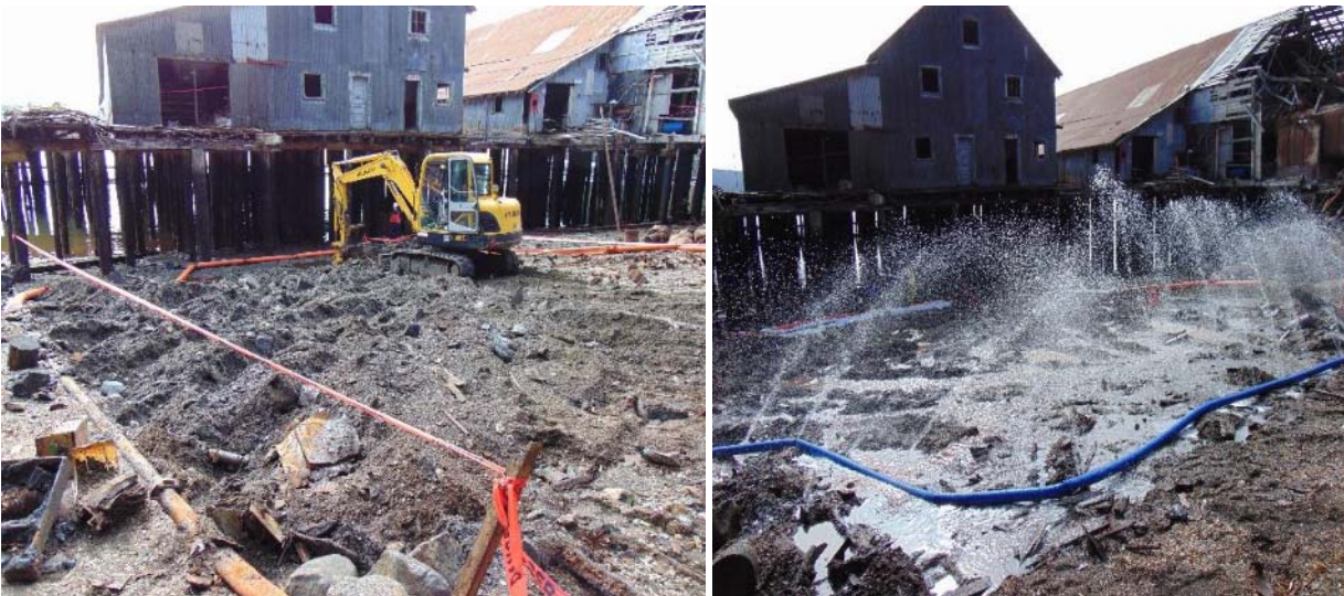
Photo of beach tilling and deluge. Taken April 5 to 7, 2018. Photo credit: Alaska Chadux Corporation
