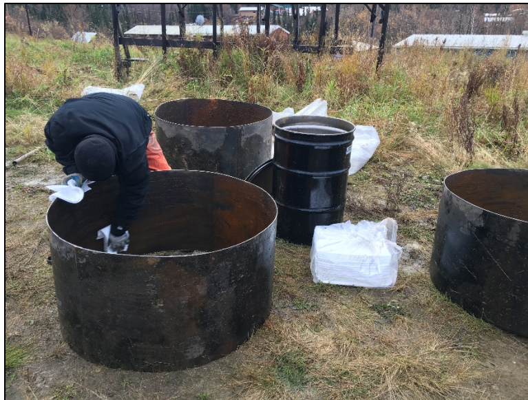
Photo 18. Final cleaning of tank sections to be recycled as fire pits.
