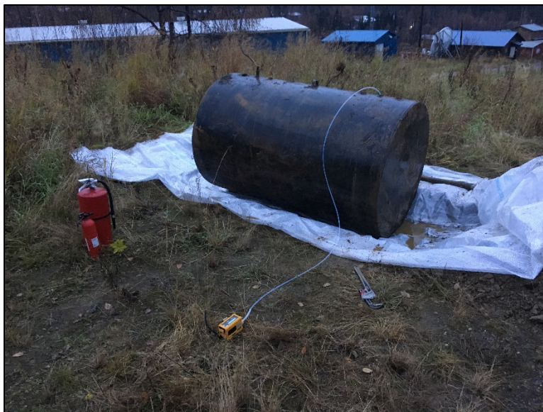
Photo 14. Gas monitoring of tank interior prior to cutting.
