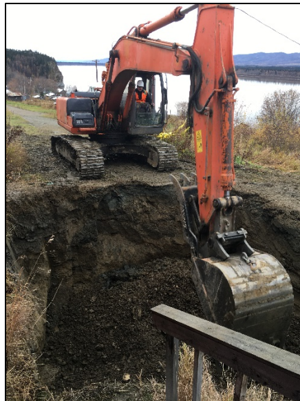
Photo 10. Spreading and compacting gravel backfill in UST area excavation.
