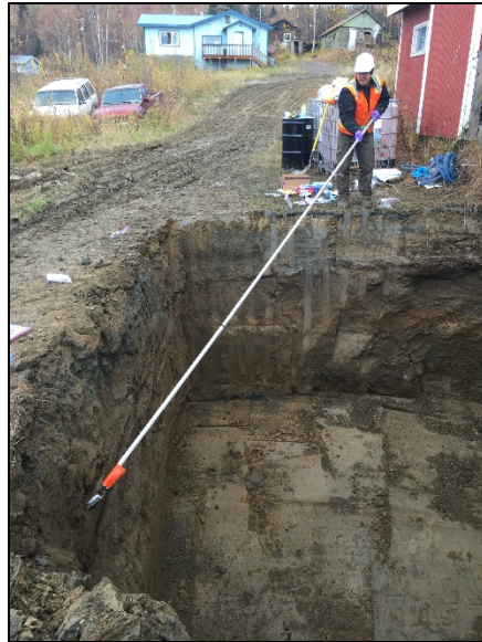
Photo 9. Collecting sidewall excavation confirmation samples using trowel extension.
