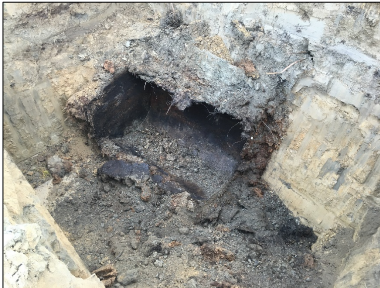
Photo 6. Excavation following tank removal. Note moss bedding around tank.
