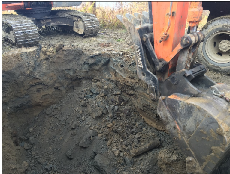
Photo 8. Removing additional soil from UST area excavation.
