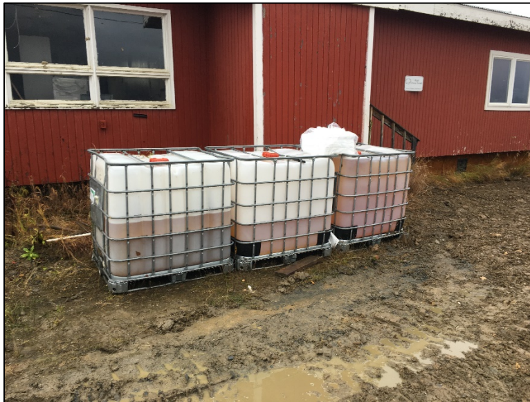
Photo 12. Liquids removed from UST. Tanks on right contain heating oil, tank on left contains a mix of oil and water.
