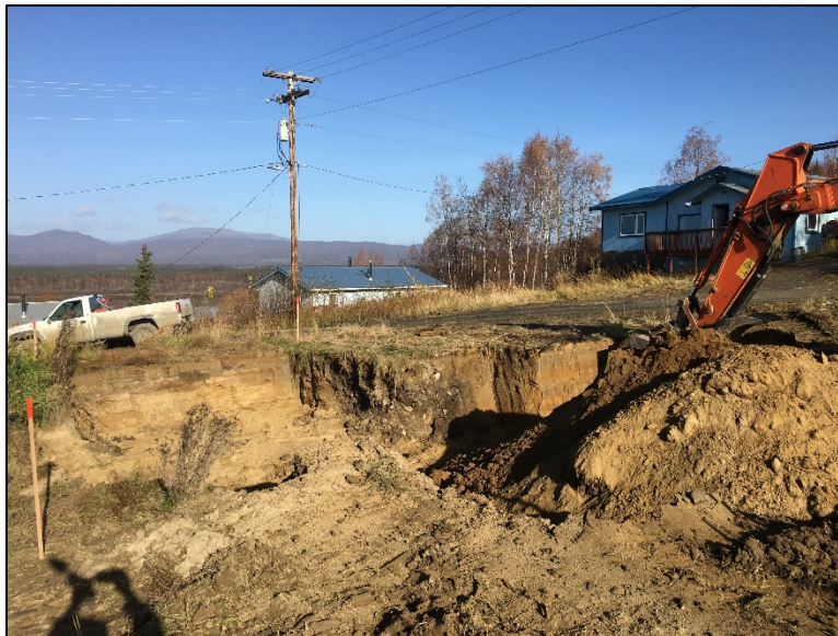
Photo 26. Removing additional soil from excavation.
