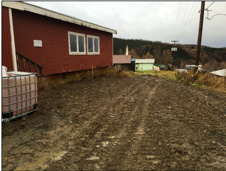
Photo 11. Finished grade following backfill (prior to final compaction).
