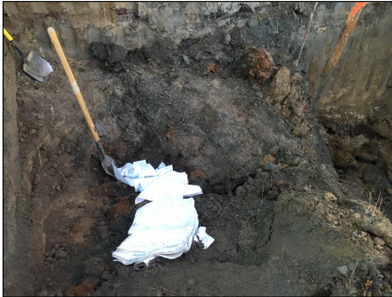
Photo 3. Second fill/vent opening in tank uncovered during hand-excavation.
