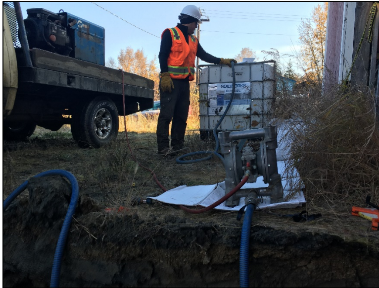
Photo 5. Transferring heating oil from UST to IBC tanks.
