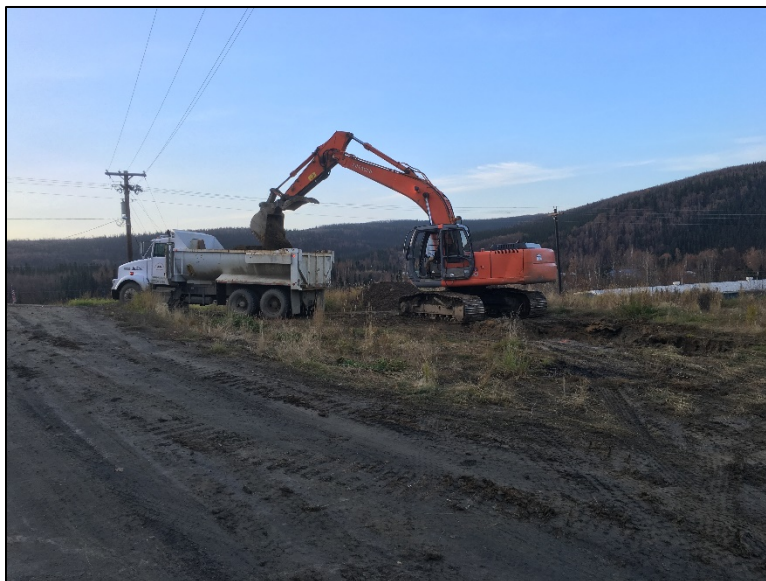
Photo 23. Starting AST-area excavation.
