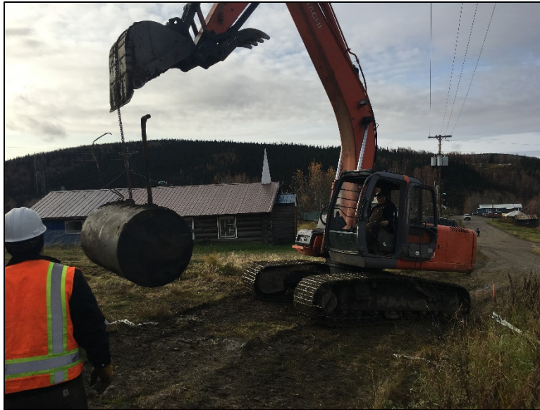
Photo 7. UST removed and transported for temporary on-site storage.
