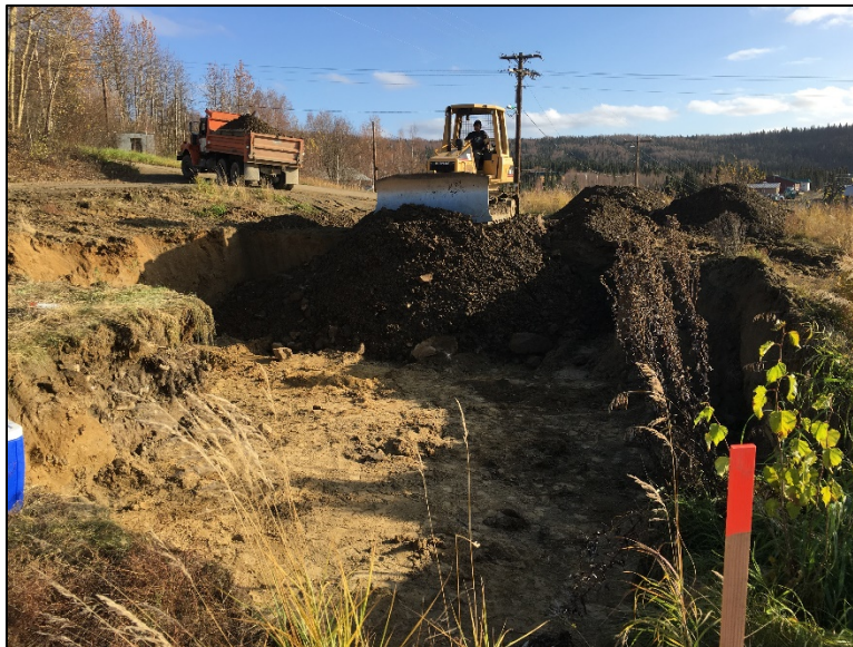
Photo 28. Backfilling AST area excavation.
