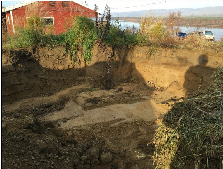
Photo 25. AST area excavation completed to 4 foot depth (still numerous hot spots at excavation floor).
