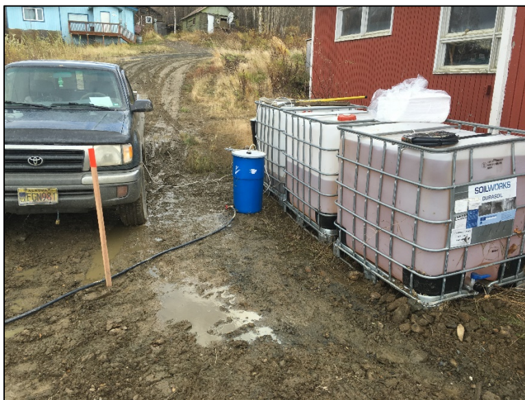
Photo 20. On-site treatment of UST water via granular activated carbon filtration.
