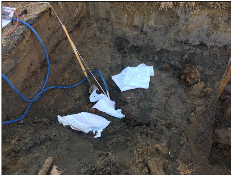
Photo 4. Liquids being pumped from the tank. Interface probe used to monitor oil-water interface.
