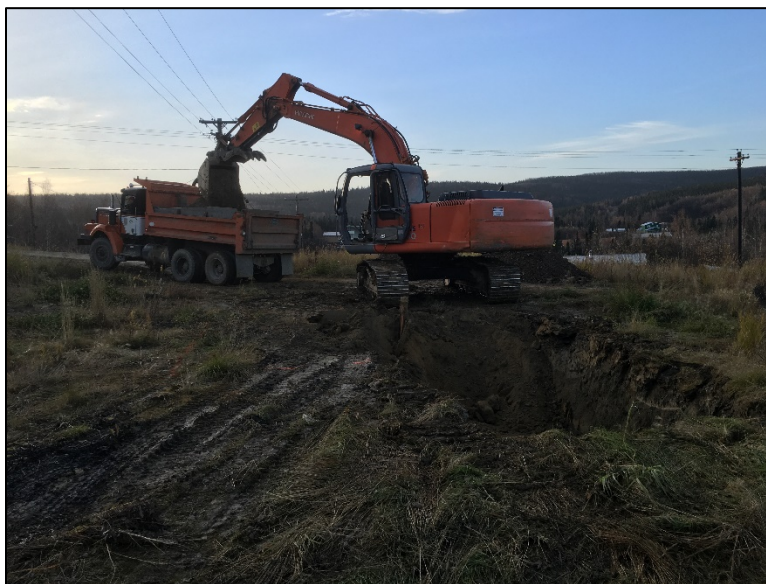
Photo 24. AST-area excavation. Note treated timber in excavation near excavator track.
