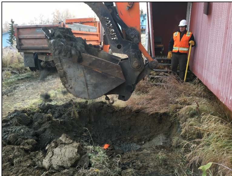
Photo 2. Beginning excavation at UST location.
