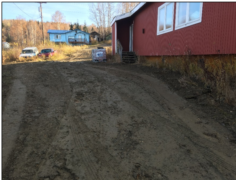
Photo 30. Finished grade, UST area, following final compaction.
