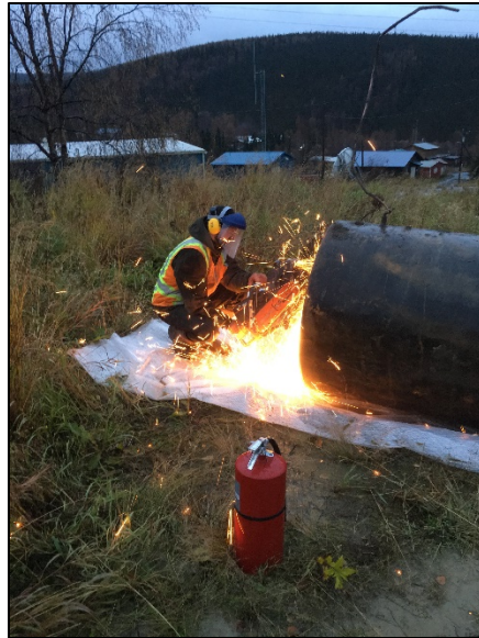
Photo 15. Cutting opening in end of tank.
