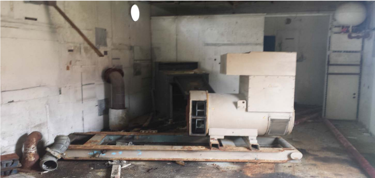
Photograph 3 – Inside the former generator building.
