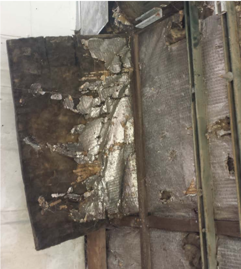
Photograph 4 – Exposed insulation in the former generator building.
