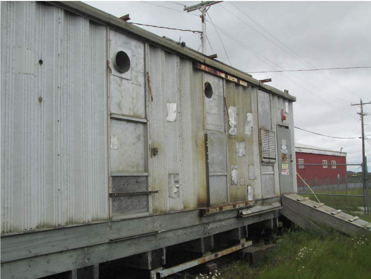
Photograph 2 – Former generator building located on the property.
