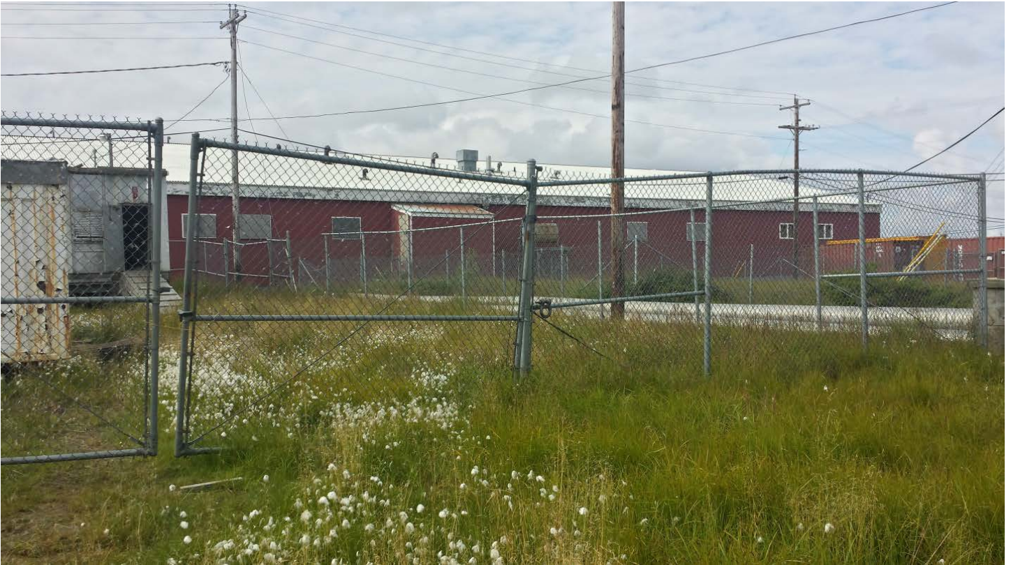
Photograph 7 – Abandoned BIA school complex from the southeast corner of the property.
