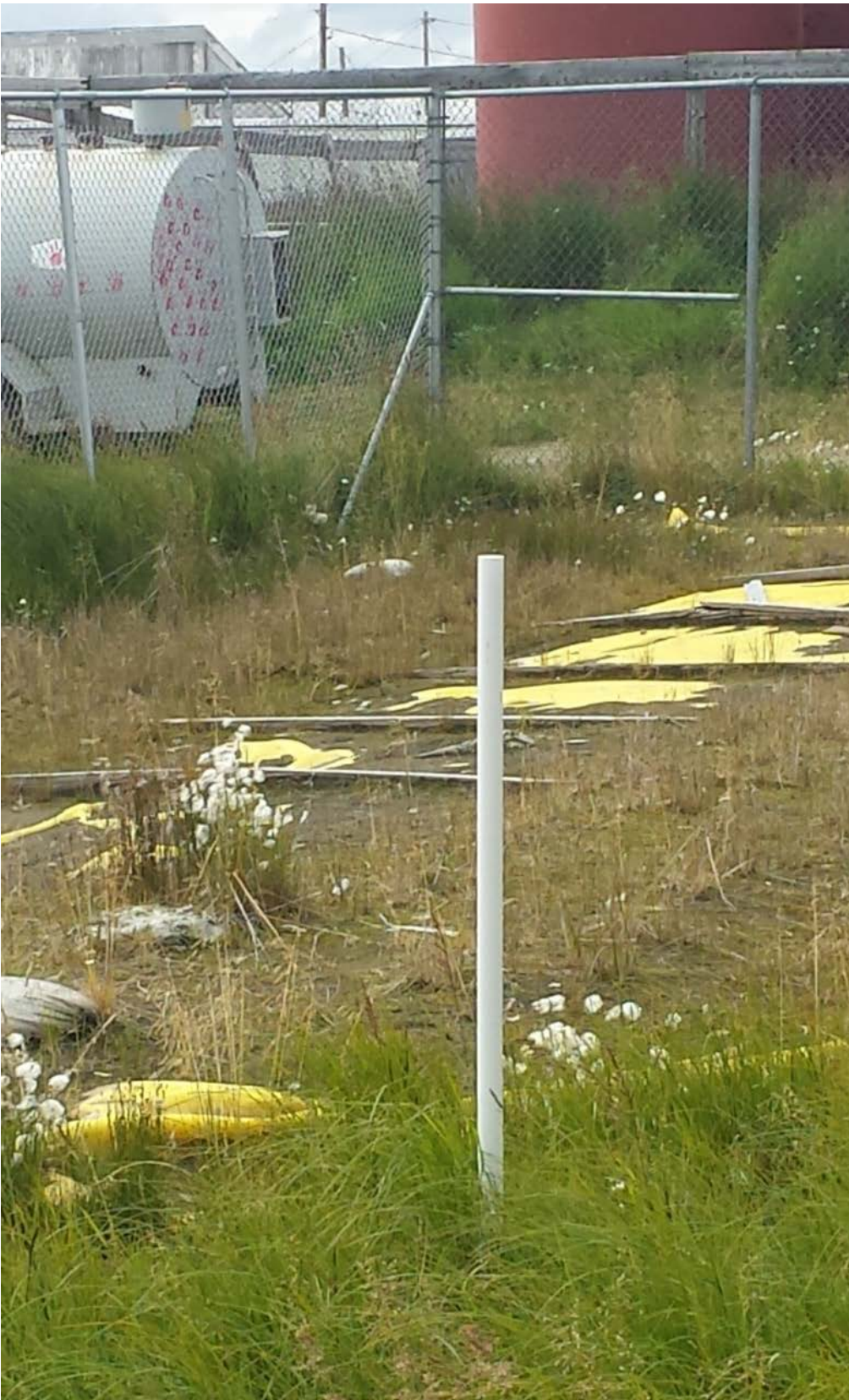
Photograph 14 – Site of a former 5,000 gallon diesel tank removed between 2007 and 2009. An interview with Mr. Stamm of AVAC indicated that he believed the pvc to be a monitoring well.
