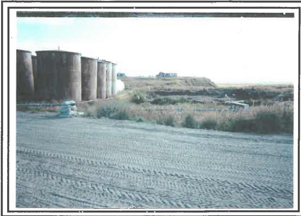
Photo 1: A view of the project site; the above ground storage tanks to the left and the bermed area to the right; looking east. (August 2002)
