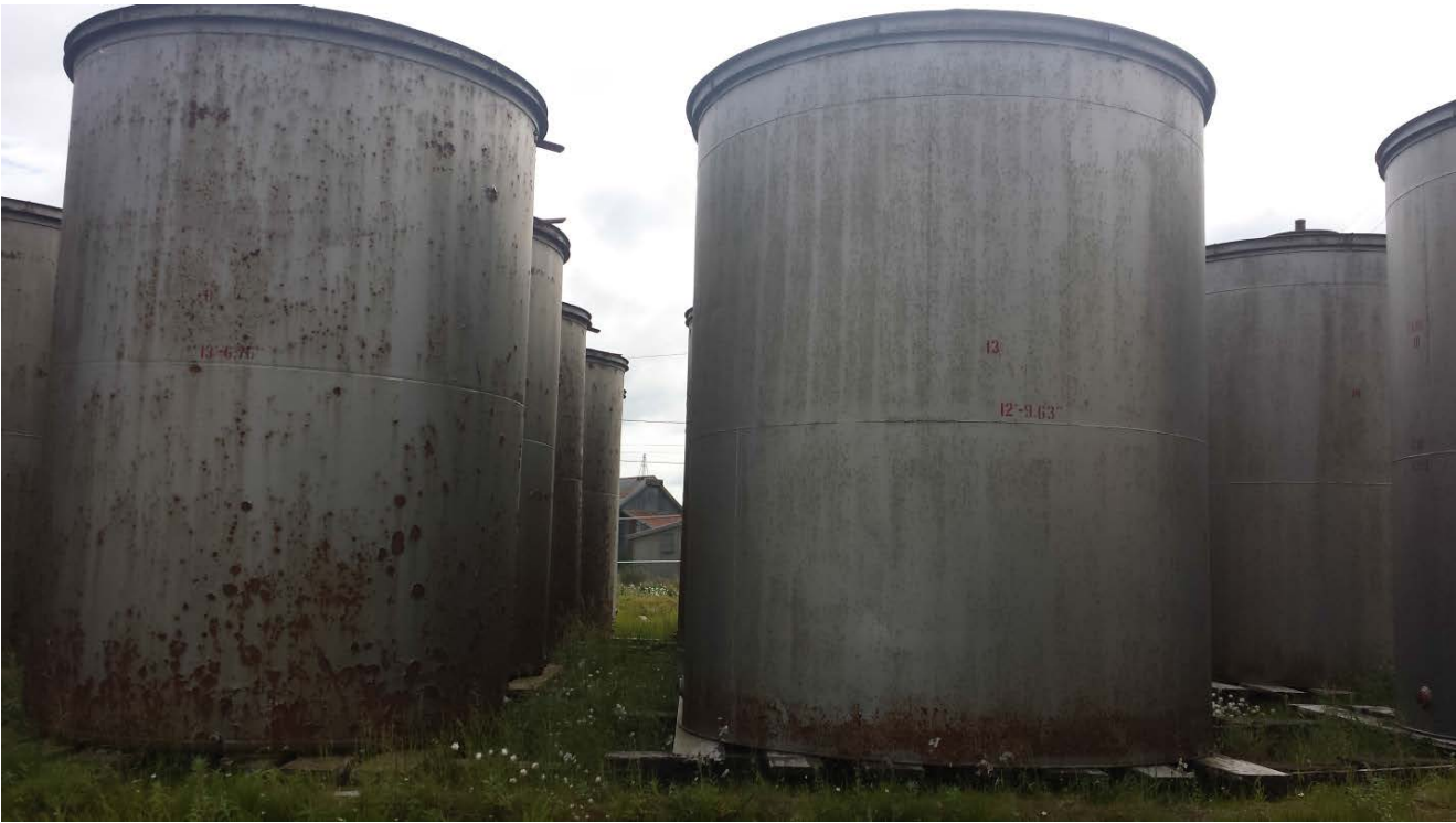
Photograph 1 – The tank farm ASTs located on the property.
