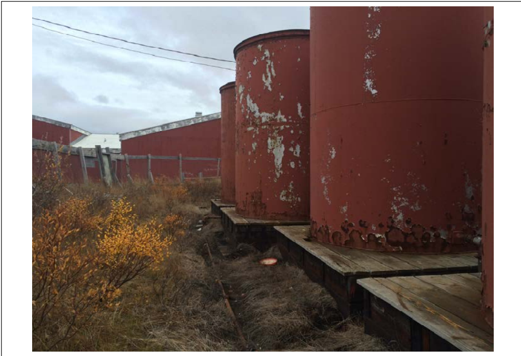
Photo 5. Stained soil along southwest edge of tank farm. Facing northwest. October 8, 2015.
