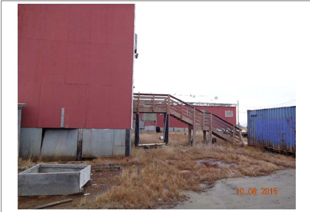
Photo 7. Southwest edge of school. Looking approximately northeast. October 8, 2015.
