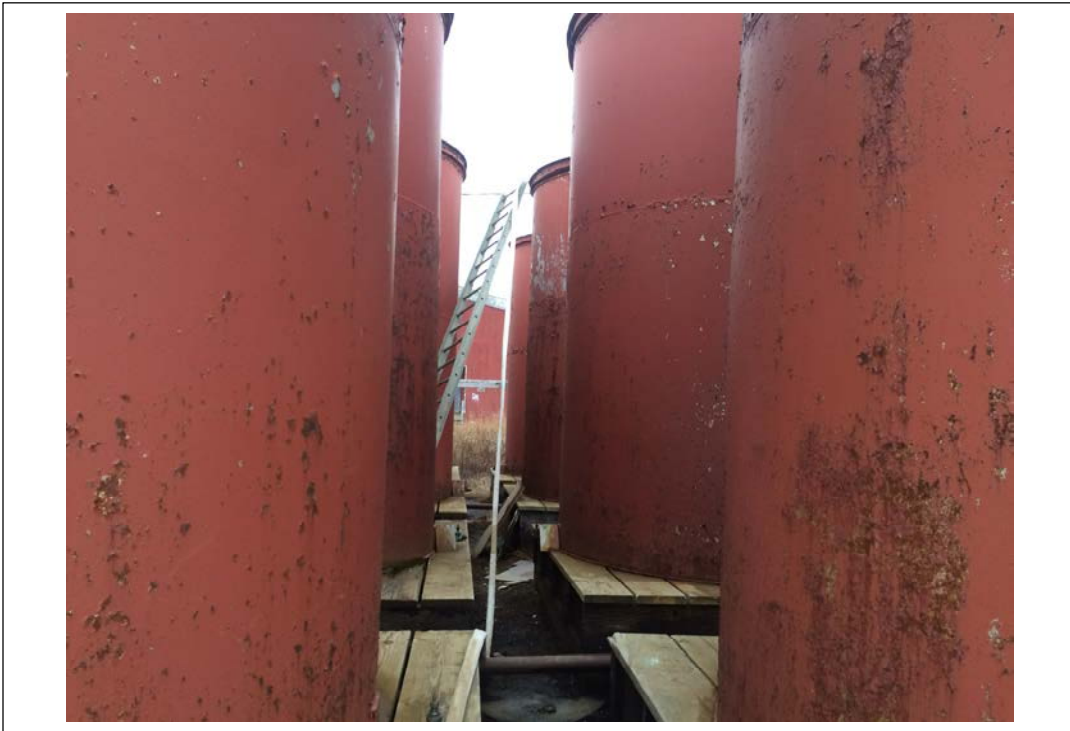
Photo 3. Hose leading to tank next to ladder. Picture taken while standing on southeast edge of tank farm. Looking northwest. October 8, 2015.
