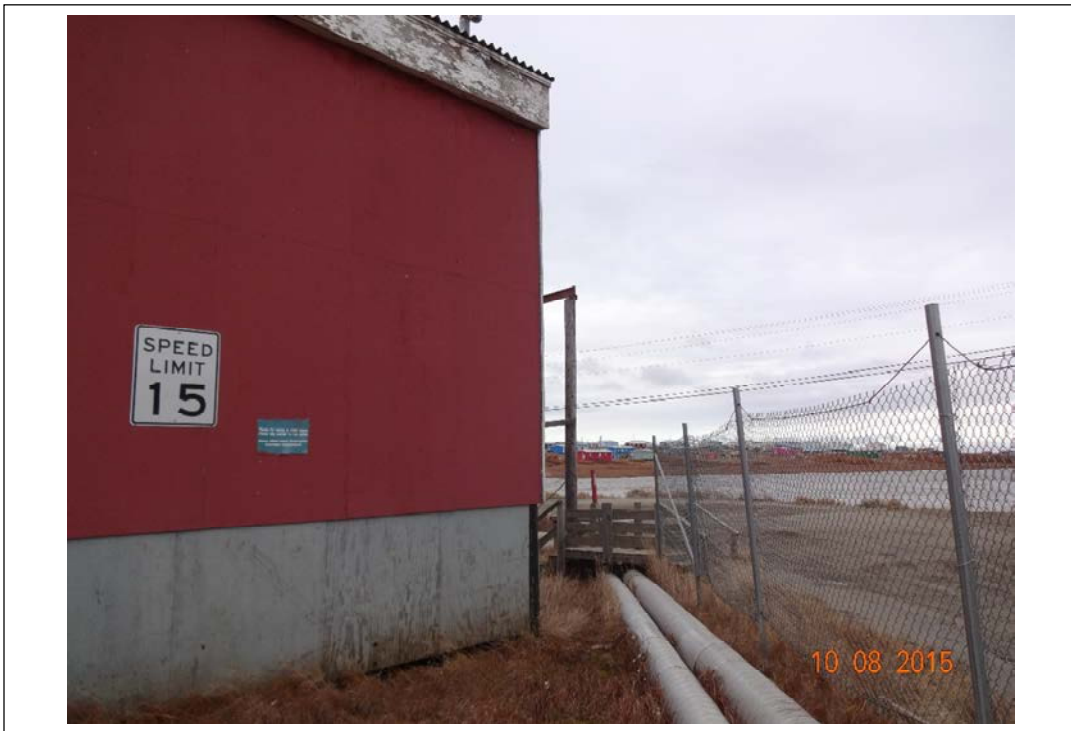
Photo 23. Northeast corner of school. Looking approximately south. October 8, 2015.
