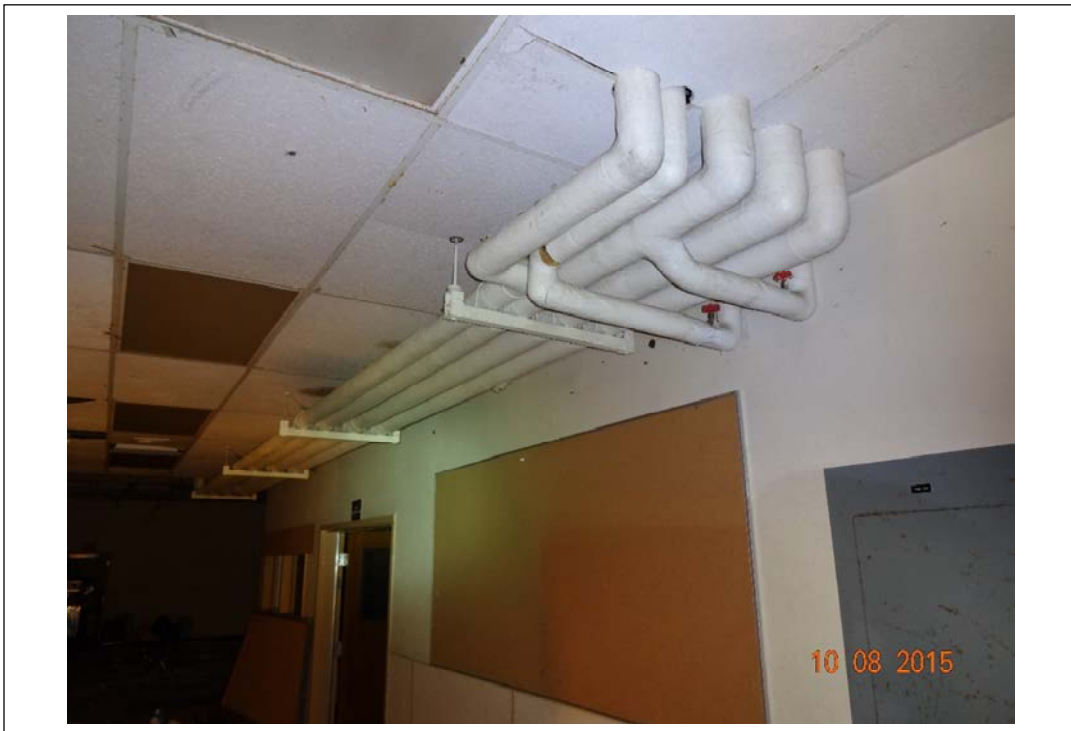
Photo 3. Possible asbestos-containing material on pipes in hallway between gymnasium and cafeteria. October 8, 2015.
