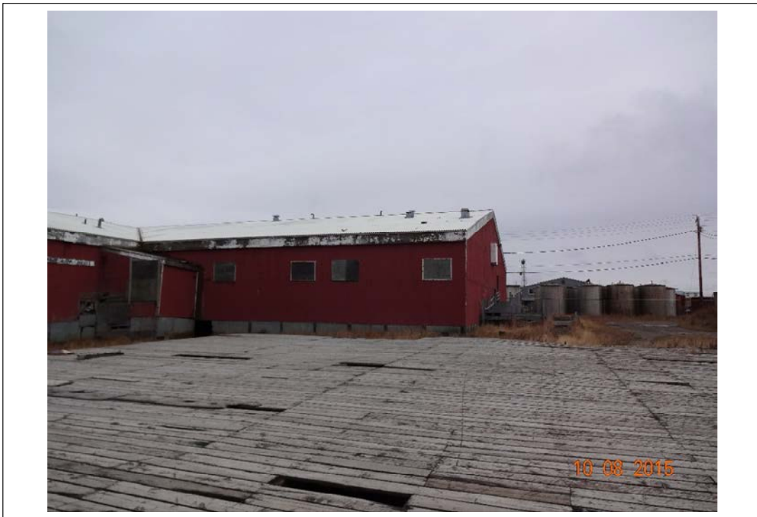
Photo 11. South corner of school. Looking approximately north. October 8, 2015.
