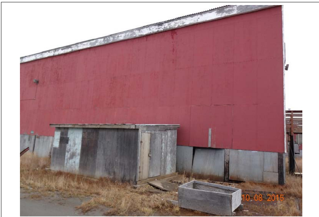
Photo 6. Southwest edge of school. Looking approximately northeast. October 8, 2015.
