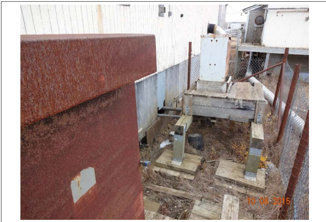
Photo 31. Transformer 1 on left, Transformer 2 on right. October 8, 2015.
