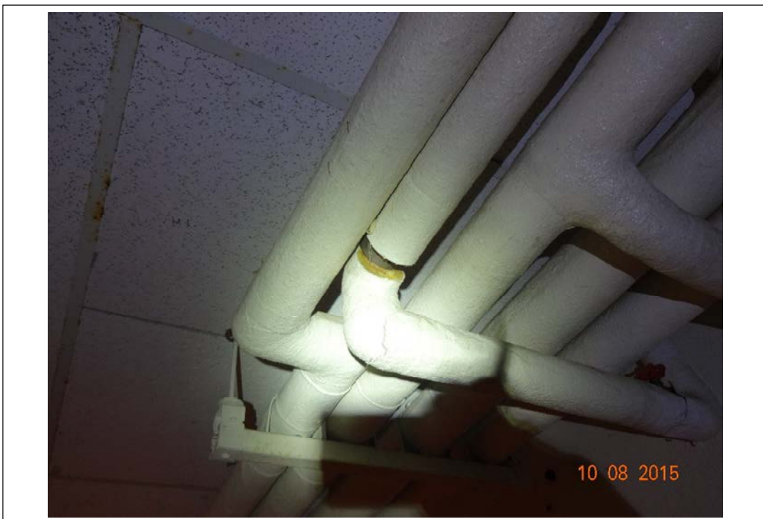
Photo 4. Possible asbestos-containing material on pipes in hallway between gymnasium and cafeteria. October 8, 2015.
