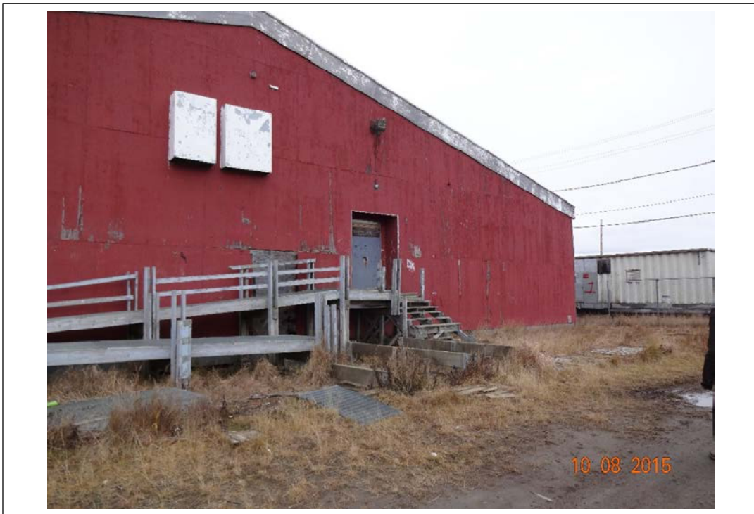
Photo 15. Southeast edge of school. Looking approximately northwest. October 8, 2015.
