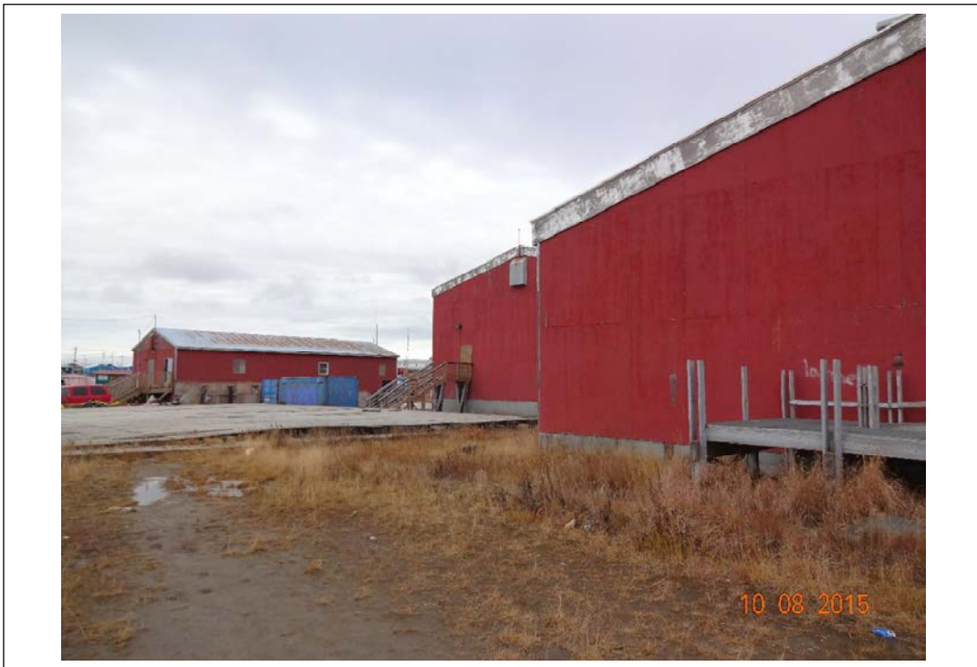
Photo 13. Southeast edge of school. Looking approximately northwest. October 8, 2015.
