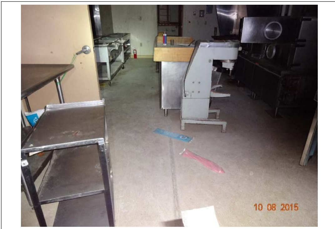
Photo 7. Asbestos-containing linoleum of Room 12. October 8, 2015.
