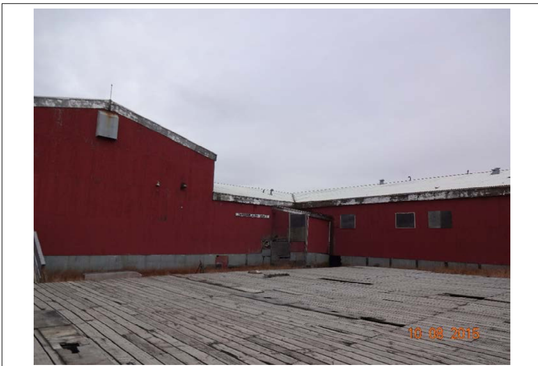
Photo 10. South corner of school. Looking approximately north. October 8, 2015.
