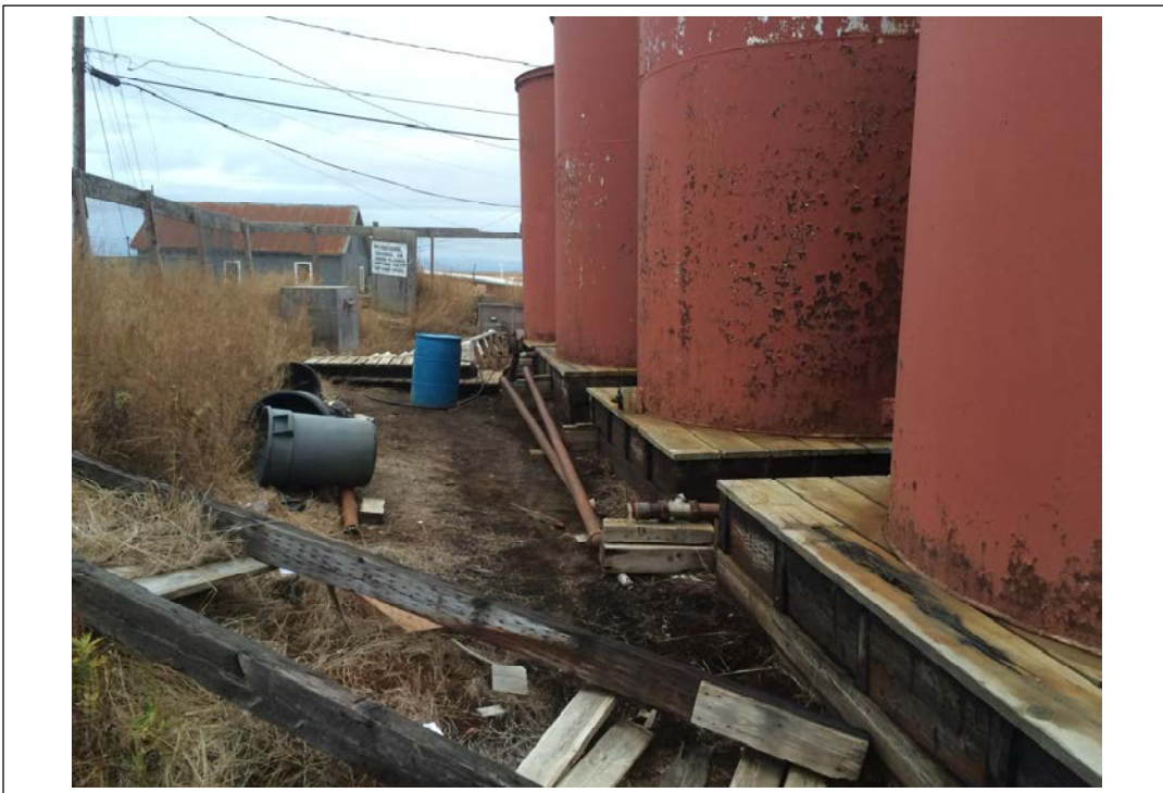
Photo 6. Stained soil and debris along northeast edge of tank farm. Looking southeast. October 8, 2015.
