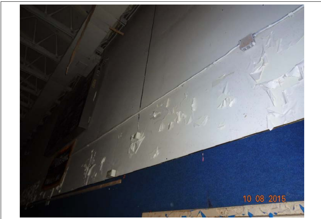
Photo 2. General interior conditions. Gymnasium. October 8, 2015.
