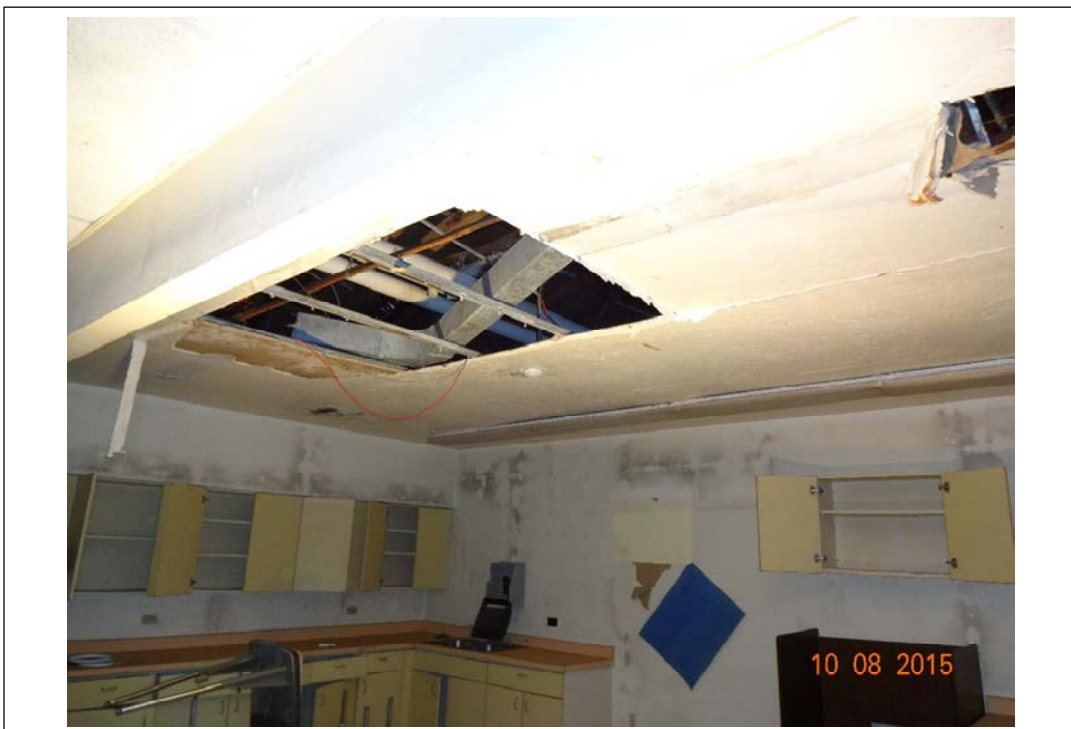
Photo 10. General interior conditions. Ceiling in Room 4. October 8, 2015.
