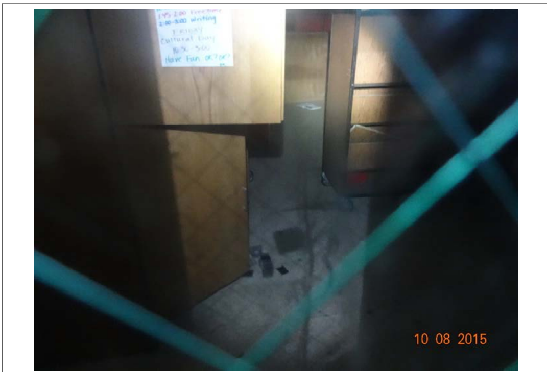
Photo 14. Asbestos-containing linoleum in Room 43. October 8, 2015.
