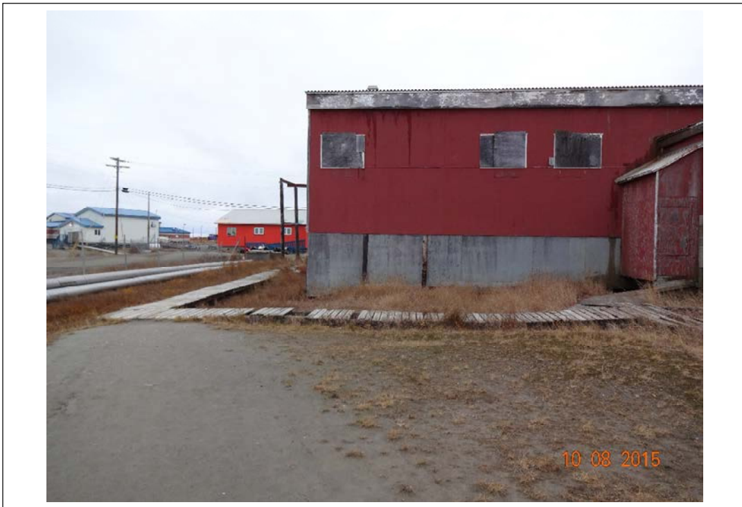
Photo 1. Northwest corner of school. Looking approximately east. October 8, 2015.
