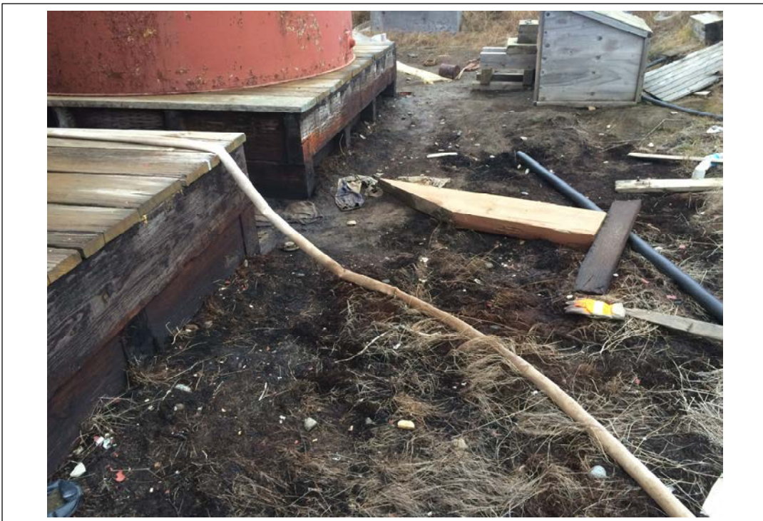
Photo 4. Same hose from Photo 3. Picture taken while standing along southeast edge of tank farm. Looking northeast. October 8, 2015.
