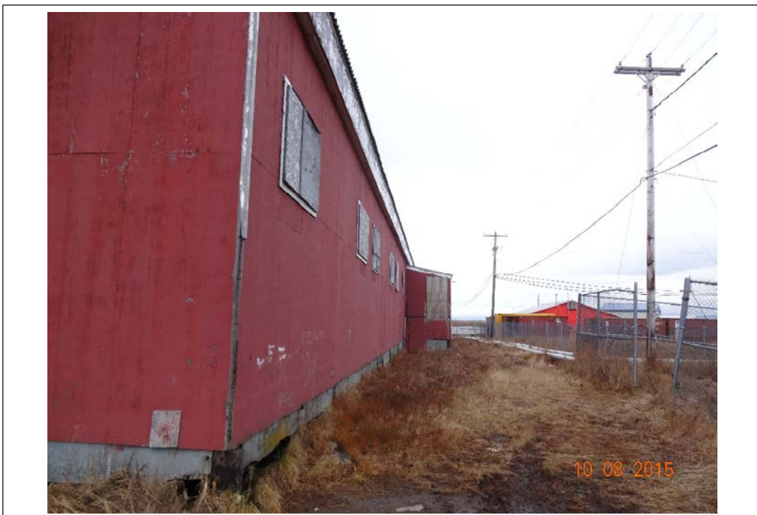
Photo 18. Southeast corner of school. Looking approximately northwest. October 8, 2015.
