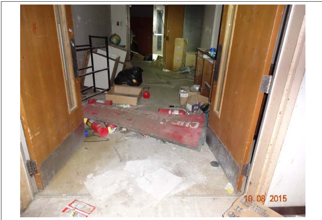
Photo 15. Asbestos-containing linoleum of Room 57. October 8, 2015.
