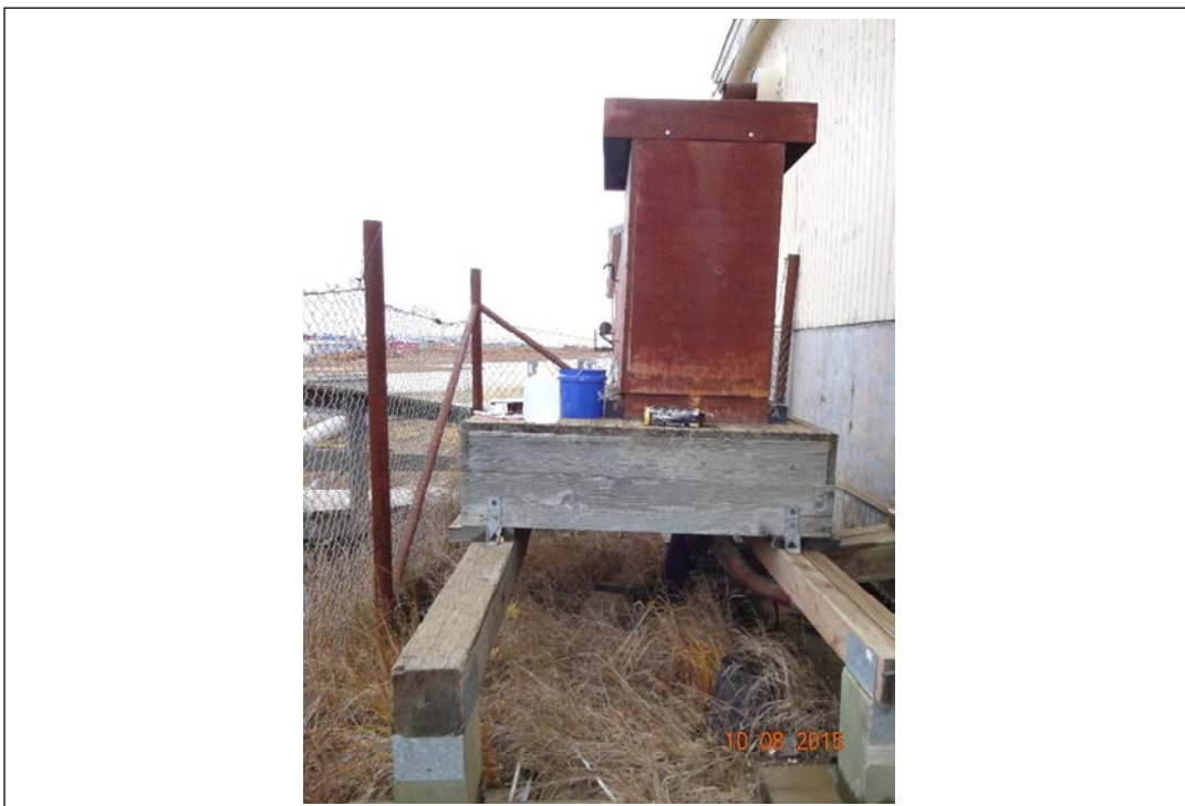
Photo 38. Location of soil sample Transformer 1: note hand auger. October 8, 2015.
