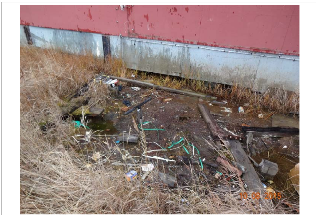
Photo 36. Location of soil sample Battery 2: note hand auger. October 8, 2015.
