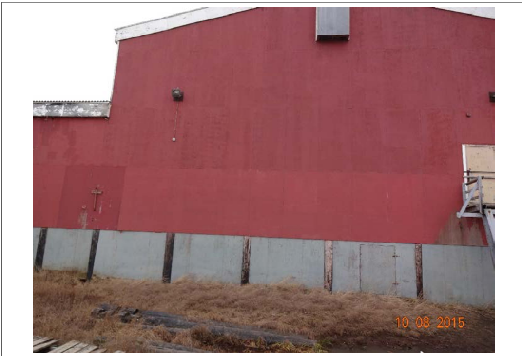
Photo 3. Northwest corner of school. Looking approximately east. October 8, 2015.
