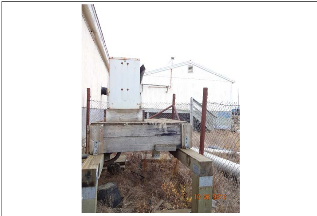
Photo 39. Location of soil sample Transformer 2: note hand auger. October 8, 2015.
