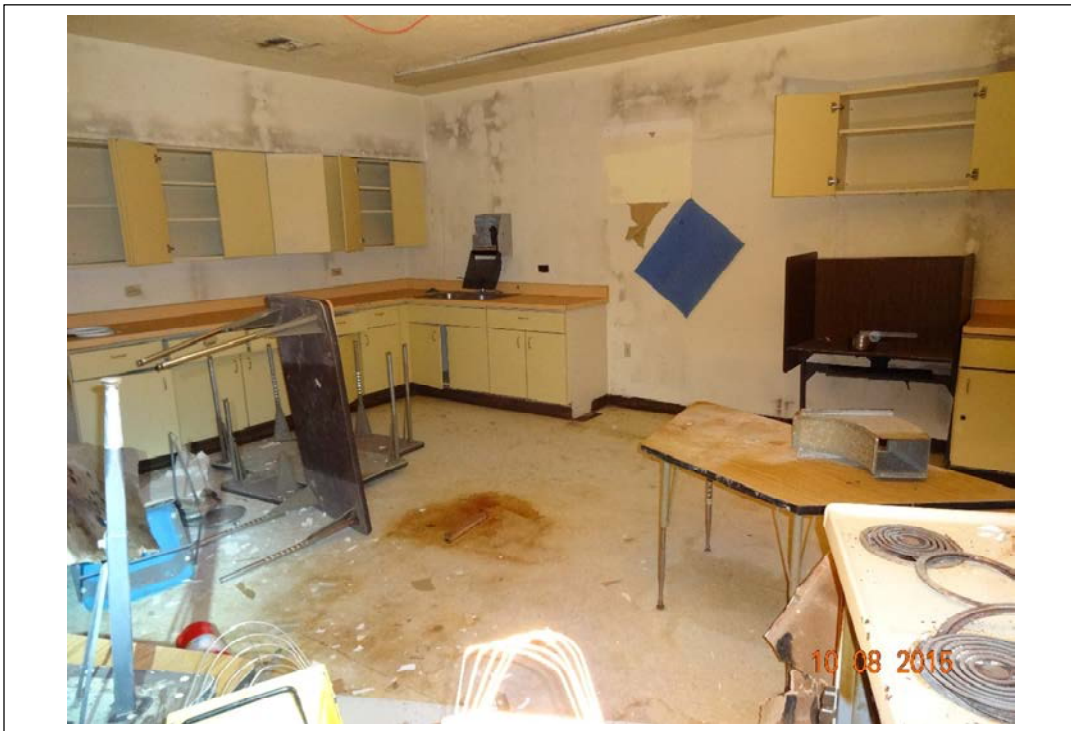
Photo 9. Asbestos-containing linoleum in Room 4. October 8, 2015.
