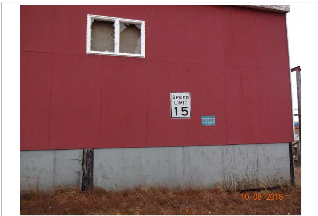
Photo 24. Northeast corner of school. Looking approximately south. October 8, 2015.
