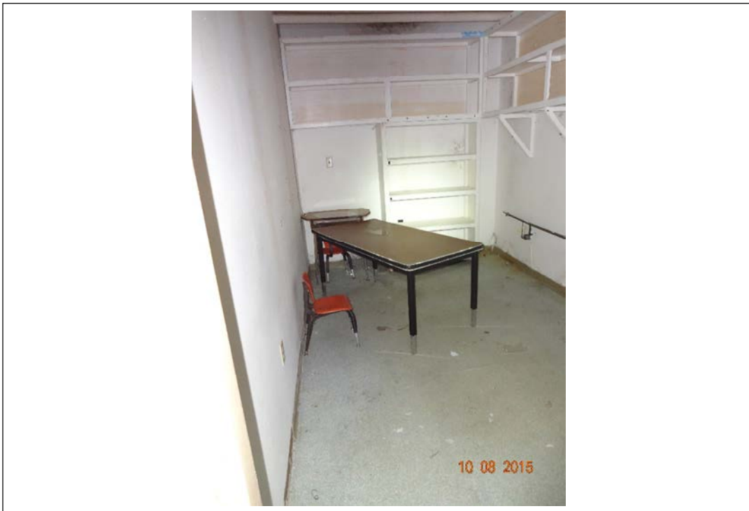
Photo 13. Asbestos-containing linoleum in Room 33 (based on map) but “13” on door. October 8, 2015.
