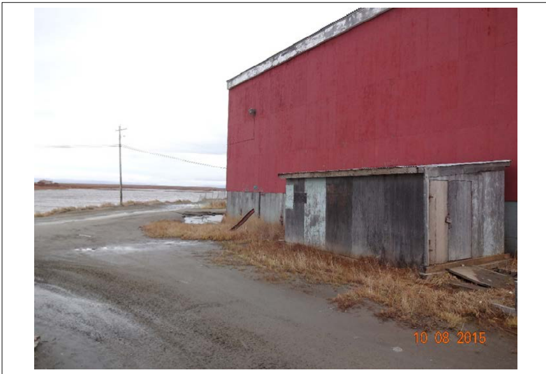
Photo 5. Southwest edge of school. Looking approximately northeast. October 8, 2015.
