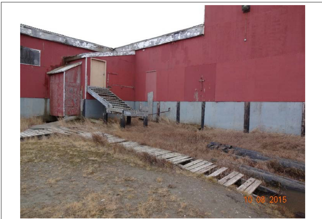
Photo 2. Northwest corner of school. Looking approximately east. October 8, 2015.
