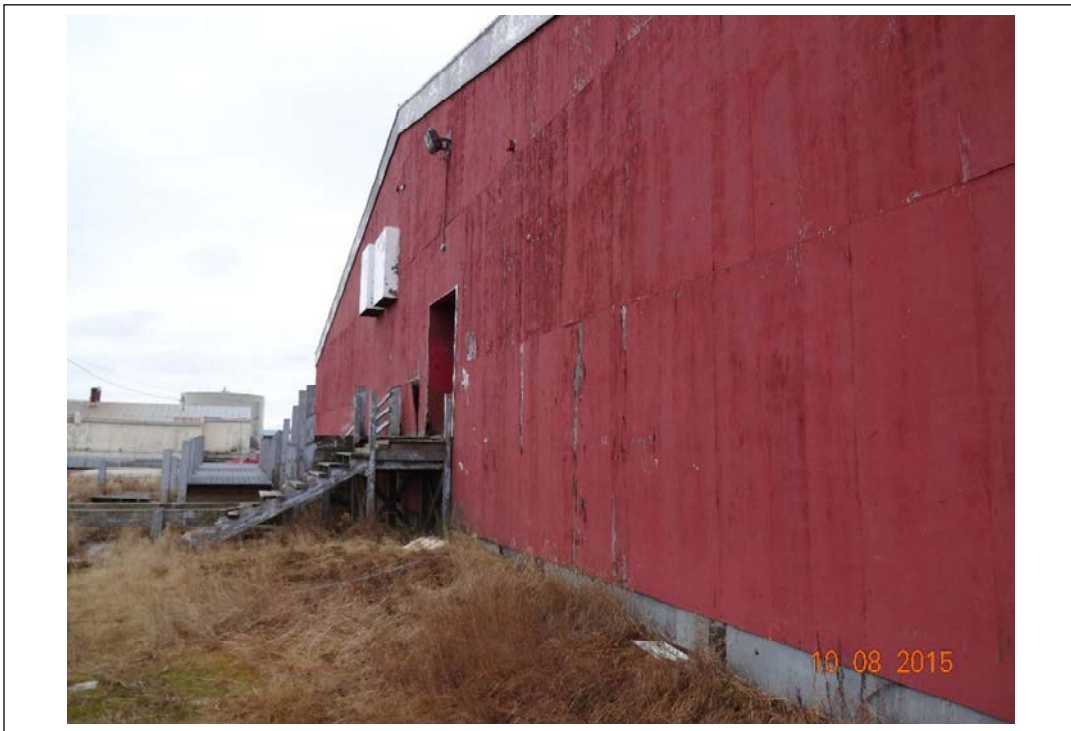
Photo 17. Southeast corner of school. Looking approximately northwest. October 8, 2015.
