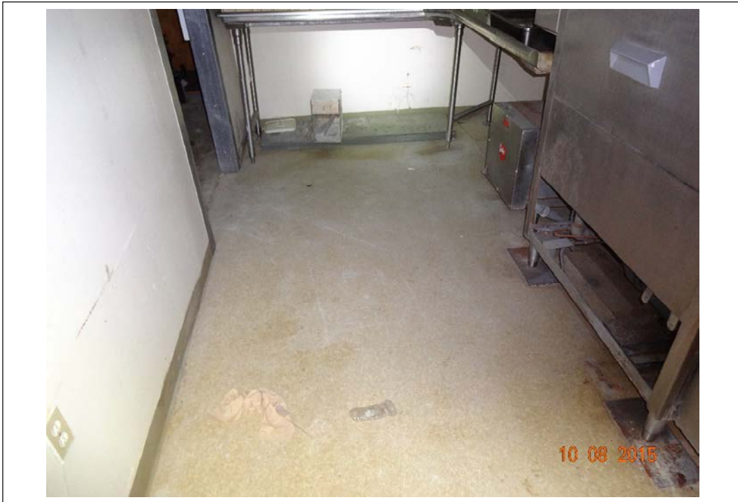
Photo 5. Asbestos-containing linoleum of Room 13. October 8, 2015.
