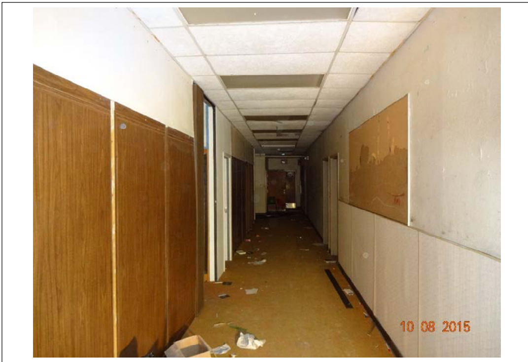
Photo 11. General interior conditions. Room 29 on left, Room 3 door just past corkboard on right. October 8, 2015.
