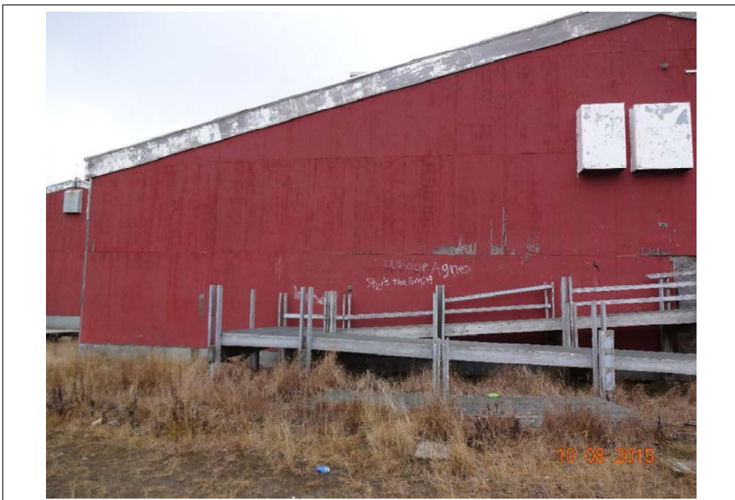
Photo 14. Southeast edge of school. Looking approximately northwest. October 8, 2015.
