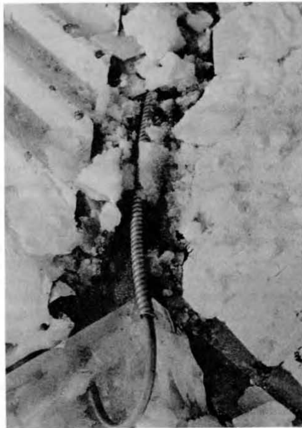
Figure 9. Electrical heat tape that has prevented the formation of slush and ice dams in the valley.
