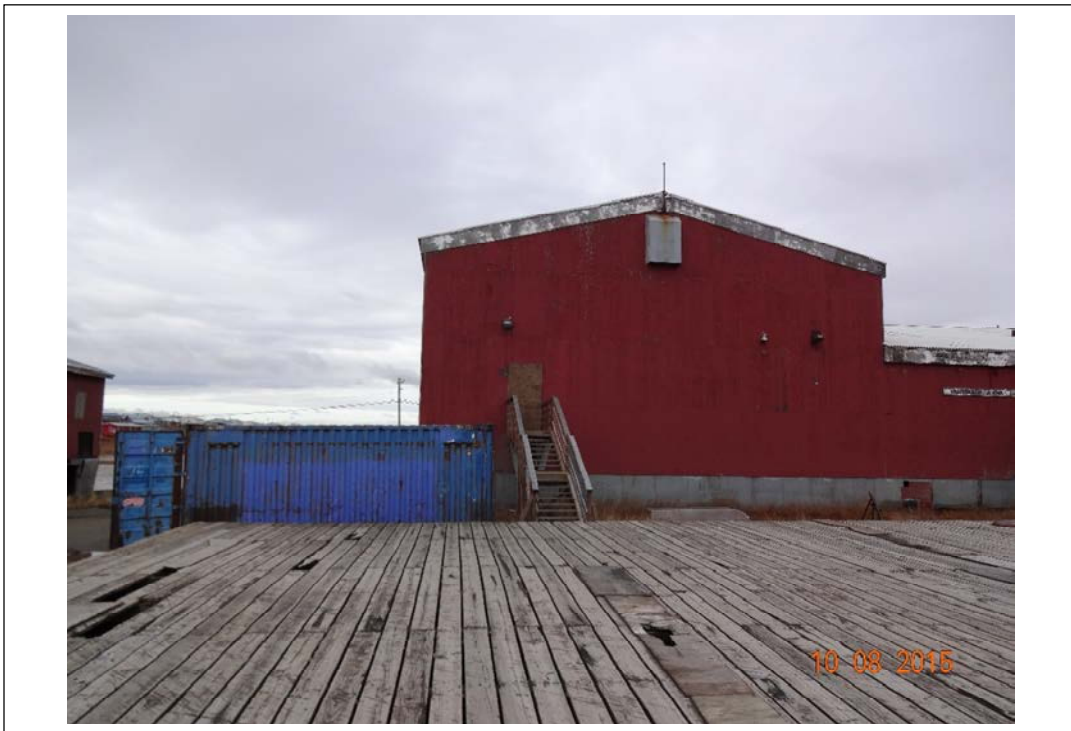
Photo 9. South corner of school. Looking approximately north. October 8, 2015.
