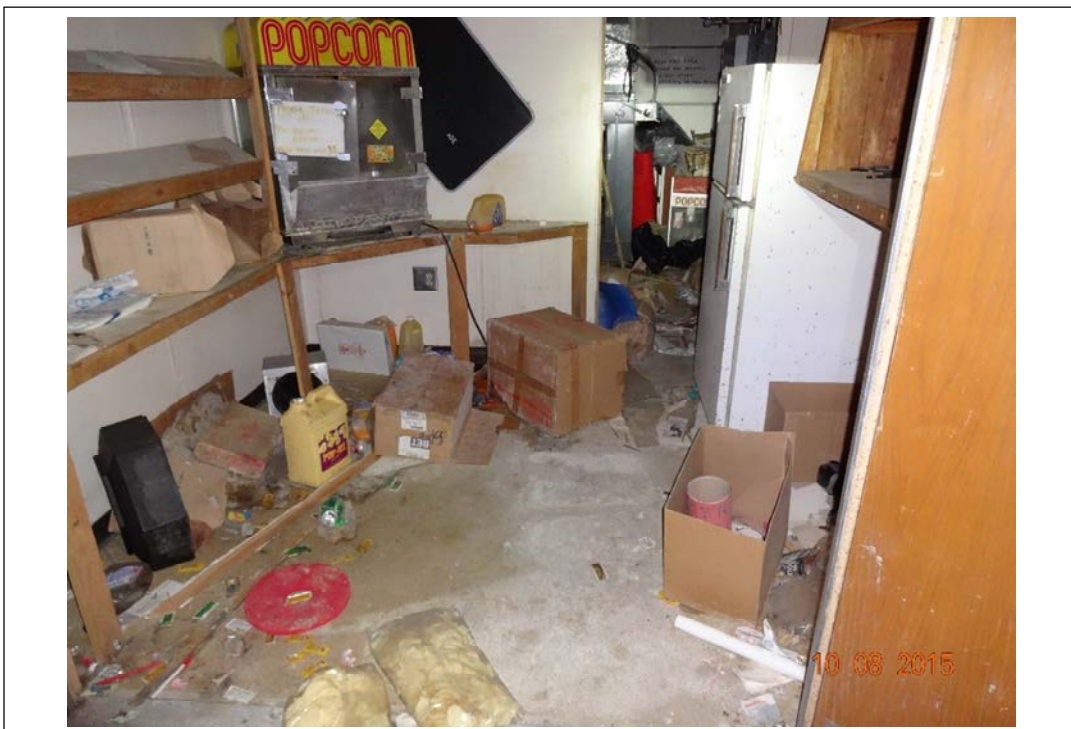
Photo 16. Asbestos-containing linoleum of Room 61. October 8, 2015.
