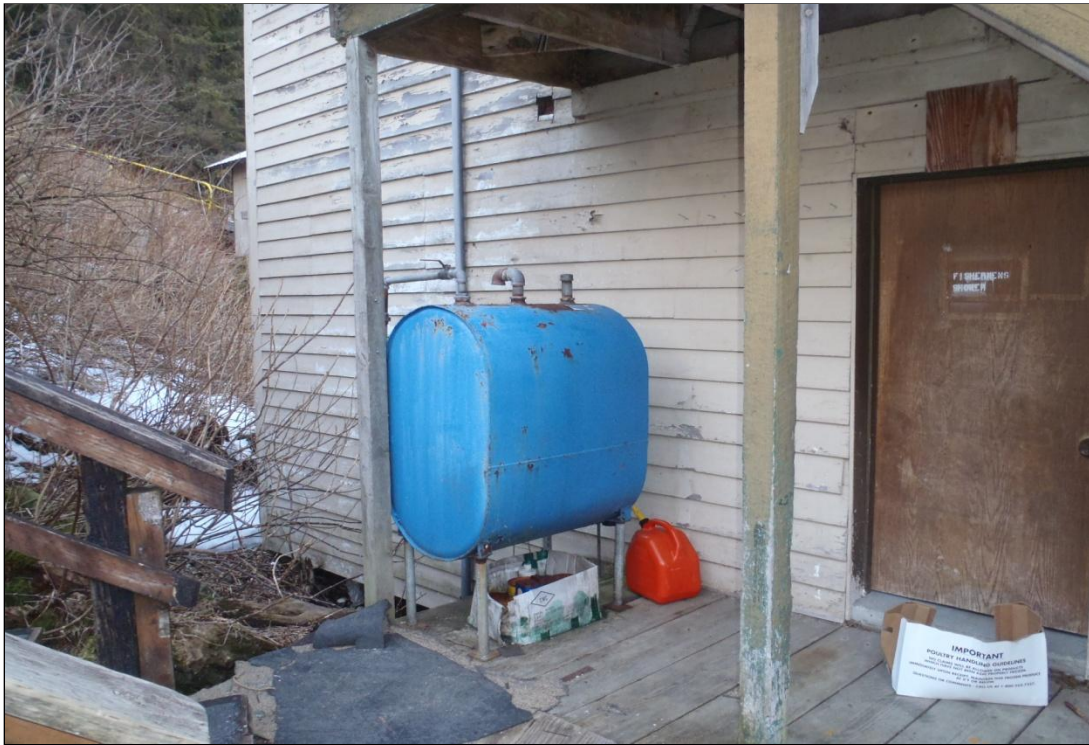
Photo 21. Heating oil AST located at southwest side of old bunkhouse.
