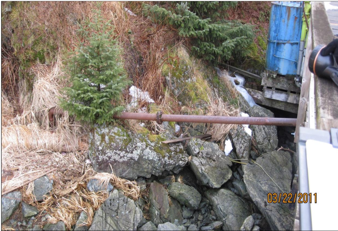
Photo 27. Unknown pipe (reportedly capped) located on the north side of boardwalk on the north side of the crab plant building.
