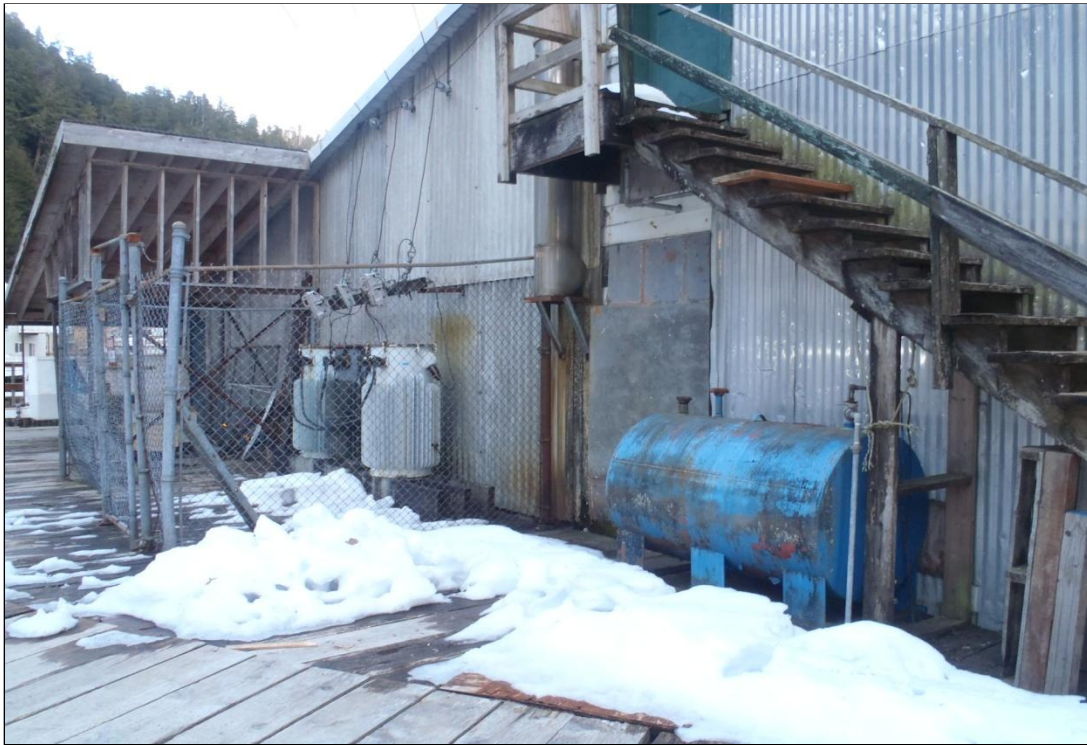
Photo 15. Heating oil AST located on the north side of the crab plant building.
