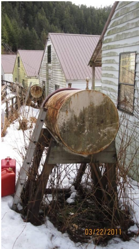
Photo 19. Company housing exterior heating oil ASTs.
