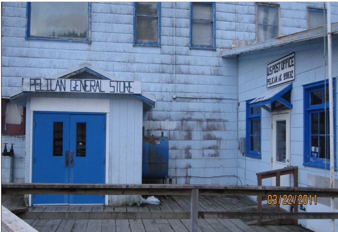
Photo 16. Heating oil AST located between the U.S. Post Office and the store.
