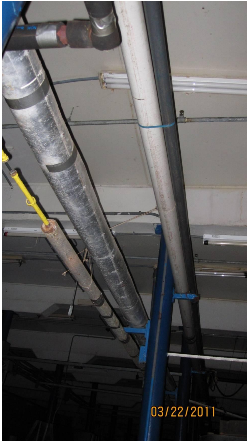
Photo 5. Potential ACM pipe insulation located on yellow pipe in photograph. Pipe is located inside crab plant building.
