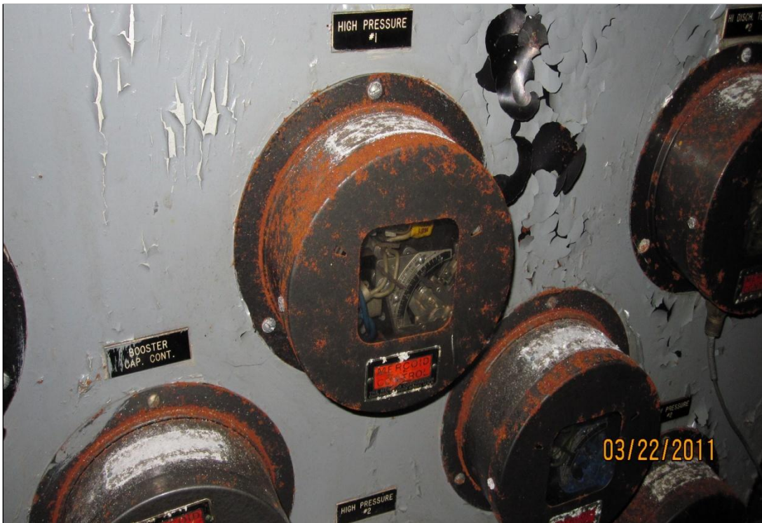
Photo 4. One of several banks of mercury switches for the ammonia refrigeration system in engine room building.
