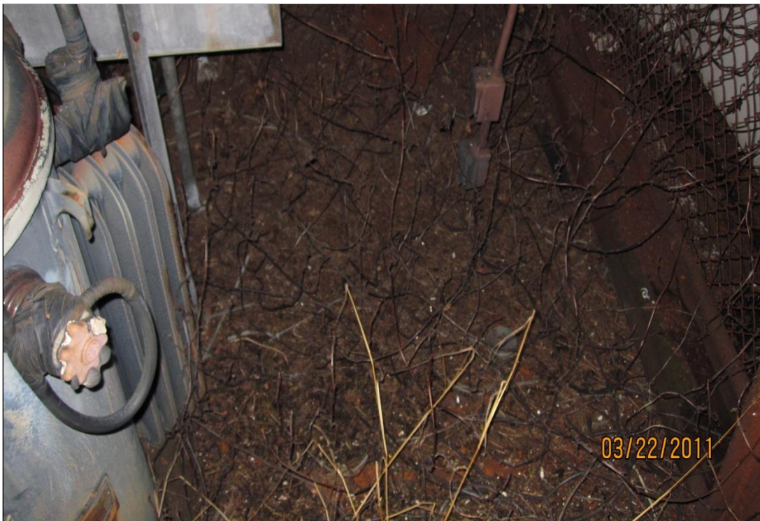
Photo 24. Discolored (stained) dirt over concrete foundation adjacent to PCB bearing transformers located on the exterior of the engine room building.
