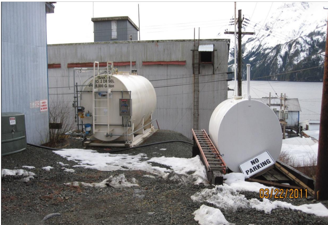
Photo 18. Power module. One of two (west most) power module 6,000 gallon ASTs, and smaller non-compliant (unplumbed) single wall AST on right side of photo.
