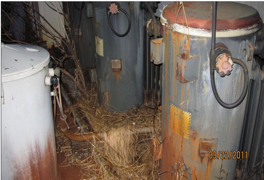
Photo 23. PCB bearing transformers located on the west exterior wall of the engine room building.
