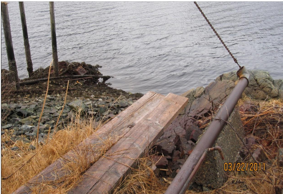
Photo 26. Discharge pipe protruding westward from engine room building. Smaller diameter pipe was reportedly used to drain oil from the ammonia compressors.
