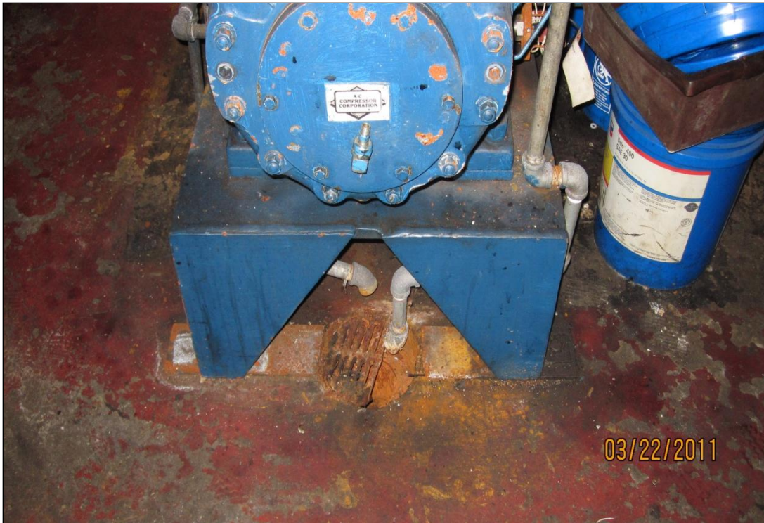
Photo 28. Floor drain located inside the engine room building. The drain is located below an ammonia compressor. Source of pipes directed towards the drain was not determined.
