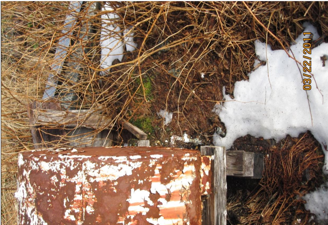
Photo 20. Easternmost company house (condemned) AST with missing pipe segment, stain, and stressed vegetation.
