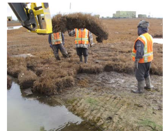
Figure 112. Moving large sod pieces
