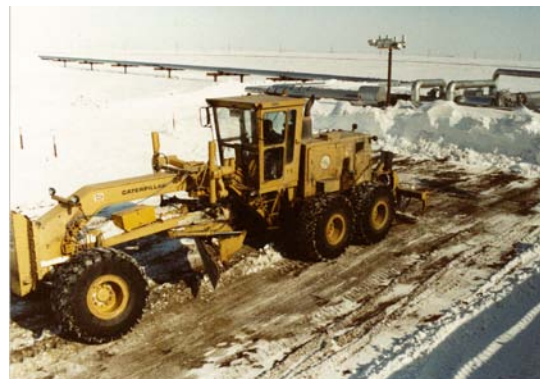
Figure 56. Scraping soil saturated with oil
