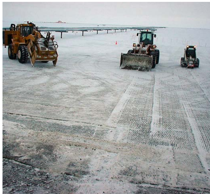
Figure 66. Site after excavation with trimmer
