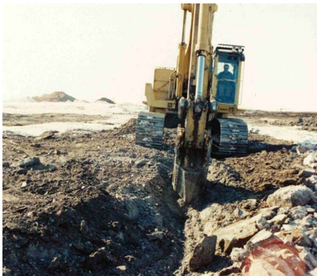
Figure 64. Backhoe excavating contaminated soil
