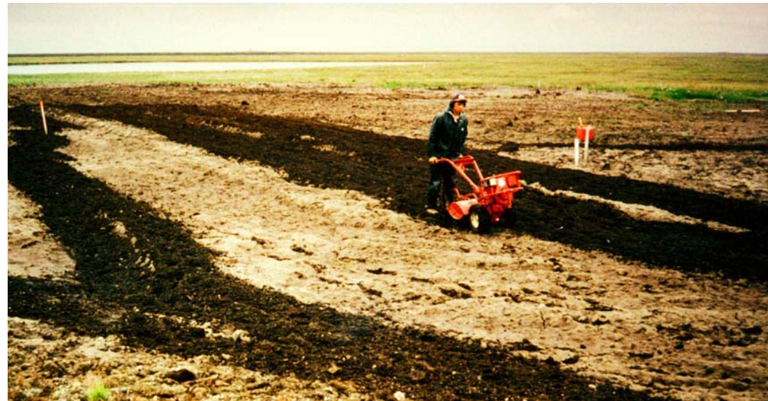
Figure 86. Rototilling contaminated soil
