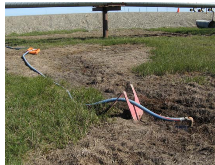
Figure 70. Natural low spot used for dewatering
