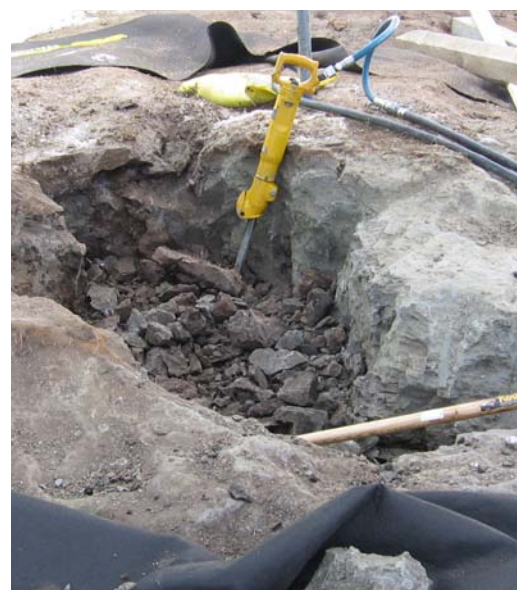
Figure 67. Excavating frozen soil with jackhammer
