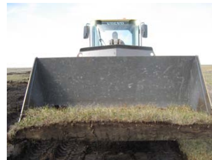
Figure 109. Intact sod harvested with a large loader
