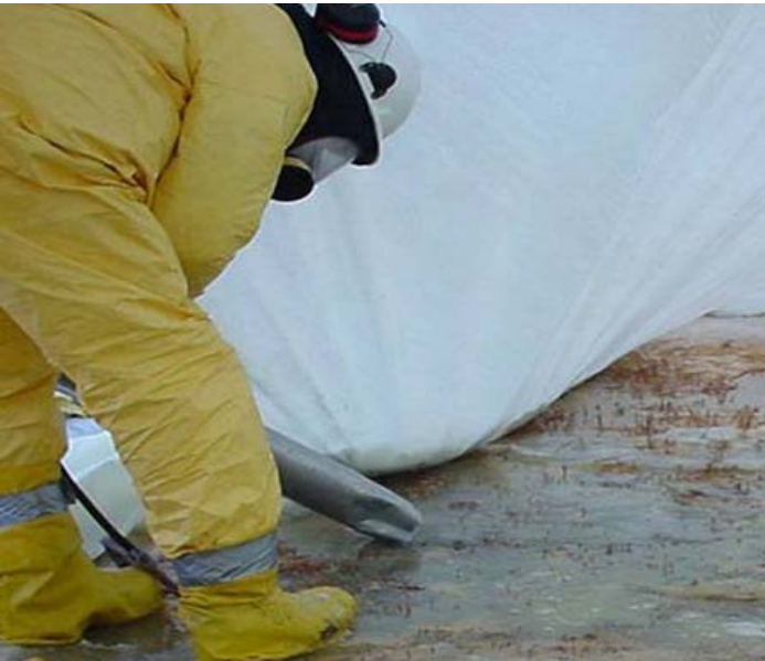
Figure 23. Vacuuming liquid contaminant
