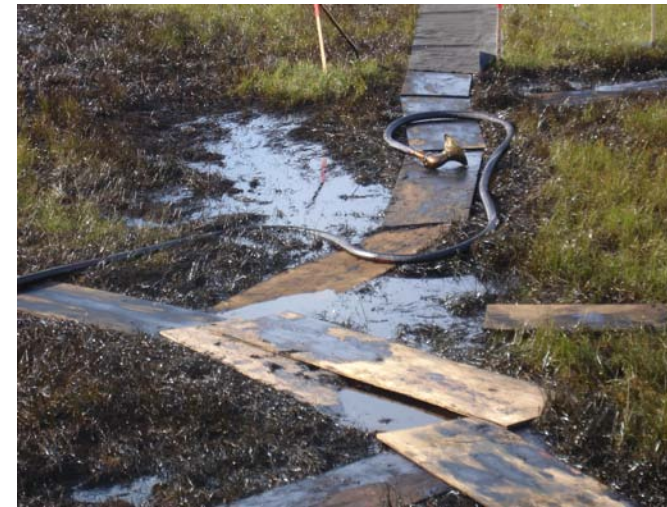
Figure 38. Vacuum hose recovering oil from low spot
