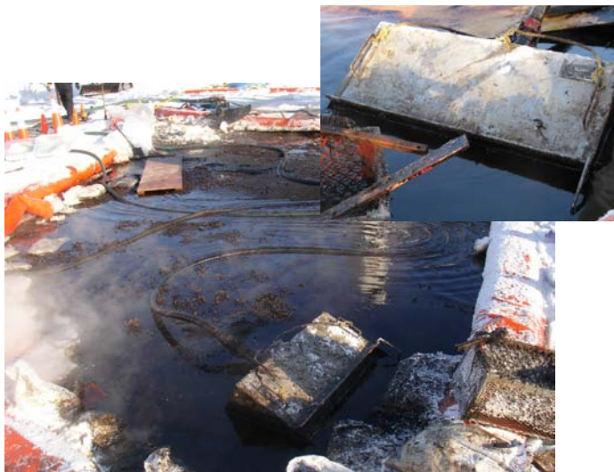
Figure 35. Skimming floating oil with slurper skimmer
