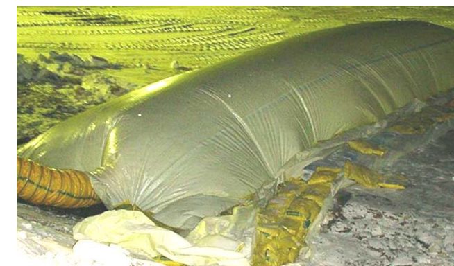
Figure 76. Heated tent to thaw soil
