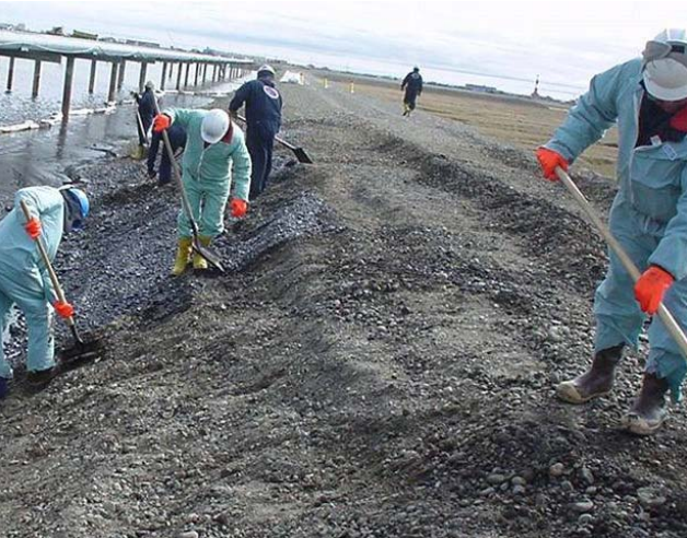
Figure 22. Shoveling contaminated gravel
