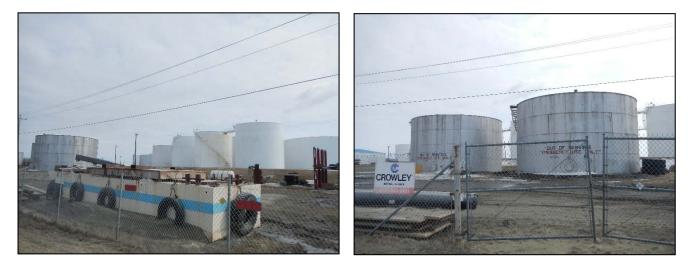
Tank Farm, 60.785458/-161.781599 (Active) – This tank farm is located south of the community, directly north of Crowley Fuel Sales. It is also owned and operated by Crowley Marine Services. It contains 5 tanks with a total storage capacity of 5,460,000 gallons of gasoline and diesel. The tank farm is within lined, secondary containment. It is approximately 740 feet from the Kuskokwim River, which has a seawall in place to prevent erosion.
