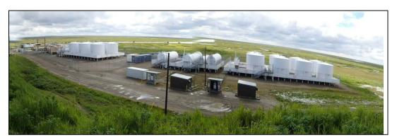
Water Treatment Plant Tanks, 61.527680/-165.589678 (Active) –This site is centrally located in town next to Chevak Lake, across from the clinic. The site was constructed around 1997 and includes four tanks that are approximately 10,000 gallons in volume. The tank farm is fully fenced and the tanks are elevated on a gravel pad with no visible secondary containment. The nearest source of erosion is the Ninglikfak River 800 feet away.
