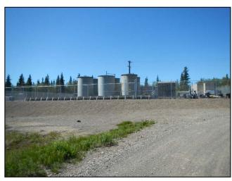
➤ City Fuel Tanks, 59.346353/-157.479275 (Active) — This site is located 85 feet from the Nushagak River at the barge landing on the south side of the community. The site includes three horizontal fuel tanks of gasoline and diesel with a total capacity of 65,000 gallons. The tanks are partially fenced and still have a new spill response kit. These tanks serve as the fueling station for the community and are operated by the City of Ekwok.
