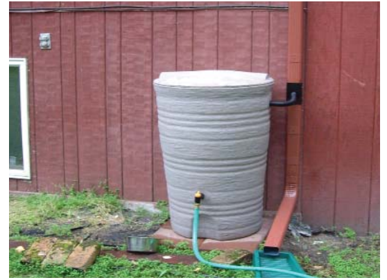
Jo Romine's Rain Barrel System
