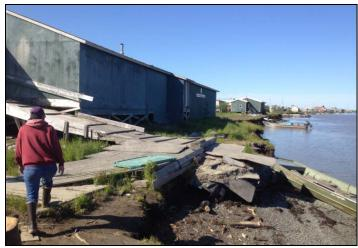
➤ Kotlik Electric Former Tank Farm, 63.032236/-163.552541 (Active) – This former tank farm is a known Contaminated Site (File ID 2423.38.002). It was the site of an approximately 7,000 gallon diesel fuel spill in 1993 with an estimated 1,000 gallons remaining after the initial cleanup. The tanks at this site have been removed and work is ongoing. The site is 445 feet from the Kotlik River.
