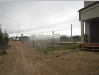
➤ Two Old Tanks, 59.109889/-156.859458 (Inactive) — This site consisted of two vertical, BIA-style tanks used for gasoline storage. It is no longer in use since the new tank farm was constructed in 2010. During the site visit a fuel odor was observed. Standing water within the secondary containment produced sheen when mixed. Tanks were labeled 'Out of Service'. This site is located approximately 65 feet from the eroding bluff of the Kvichak River.
