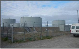
➤ Fueling Station Tank Farm, 68.347285/-166.739909 (Active) – This tank farm is located on the southwest side of the community. It is operated by the North Slope Borough and serves as the community fueling station. The site contains two small horizontal tanks with unknown capacity in a fenced secondary containment area. There was remediation work and tank farm upgrades in process during the visit. It has been in operation since around the 1980s and is located 1,050 feet from the Chukchi Sea.
