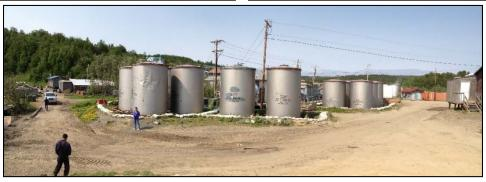
▶ BIA Tanks, 61.936812/-162.880949 (Abandoned) – This site includes three 8,740 gallon tanks on wooden pallets within an earthen berm. There is no fence to block public access. It is located 100 feet from the AVEC Tank Farm. The tanks belonged to the Bureau of Indian Affairs (BIA) School and have been in place since at least the late 1970s. They are disconnected and reported to be empty. This site lies 270 feet from the Yukon River and is within the floodline.
