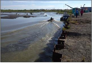
Corporation Tank Farm, 59.74499/-161.917918 (Active) – This site, owned by the Qanirtuuq Inc., contains 15 tanks of varying sizes. All tanks are within secondary containment made by a lined wooden berm. The Kanektok River and barge dock lies 170 feet away, but there is a steel corrugated wall installed for erosion mitigation at the dock.
