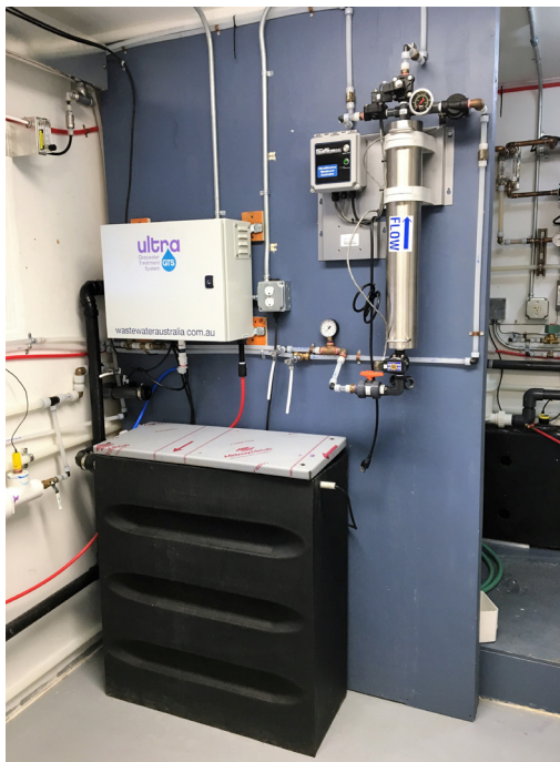
Core component of the wash water treatment system: Ultra GTS MBR tank, control panel and wash water ultrafiltration and controls.
