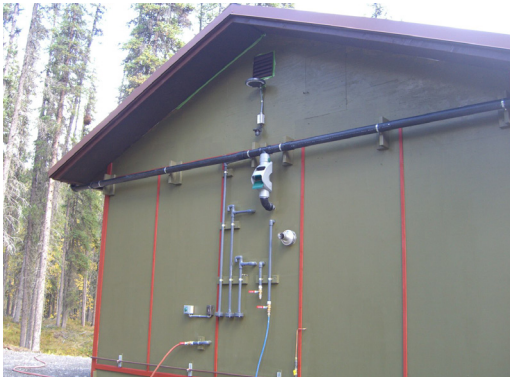
Rainwater catchment, intake and water overflow pipes, and waste water outlet.
