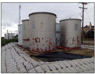
Corporation Tank Farm, 61.843567/-165.587337 (Active) – This tank farm is owned by the Askinuk Village Corporation and was constructed around 1998. It contains seventeen fuel tanks including two unused tanks. It is located on the east end of the community near the boat dock area. The site is fenced and contained within a lined, raised, earthen berm. The tanks lie within a known flooding area with the Kun River 710 feet away.
