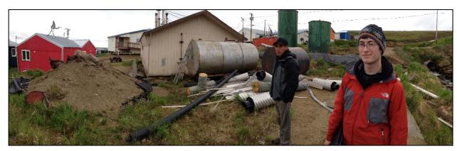
➤ Old School Tanks, 61.840728/-165.582398 (Abandoned) – This site includes three old vertical fuel tanks without secondary containment. They are are no longer in use since around 2005 when the new school was constructed. They are owned by the Lower Yukon School District. Although it is up on a hillside 2,000 feet from the Kun River, this site has erosion issues from runoff. It is 82 feet from a nearby stream.
