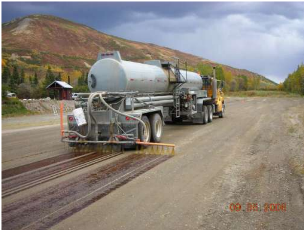
Kantishna airstrip. NPS applying EK-35 in 2006.
