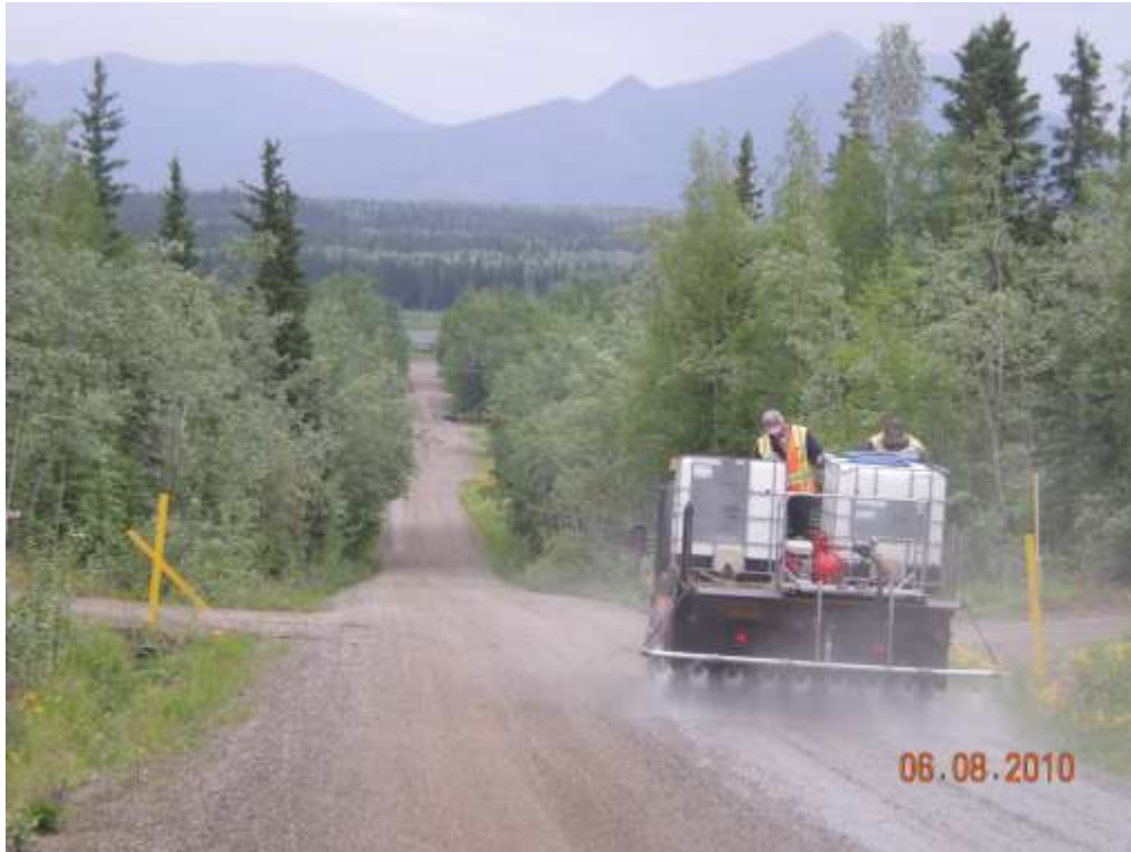
Eagle. EnviroKleen applied in spring 2010, with an "Alaska Sprayer".
