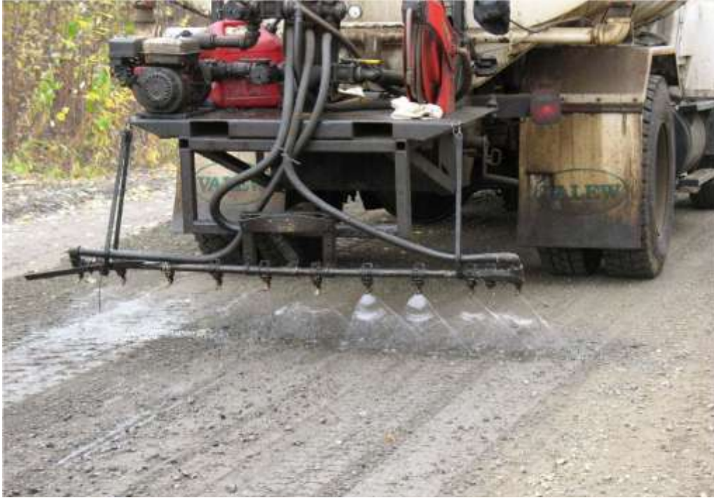
Tanana. Brice, Inc. (airport contractor) Road Work, applying Durasoil in Fall 2007.
