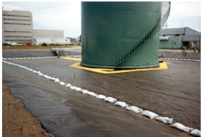
MPC Containment dike liner installation for secondary petroleum containment.
