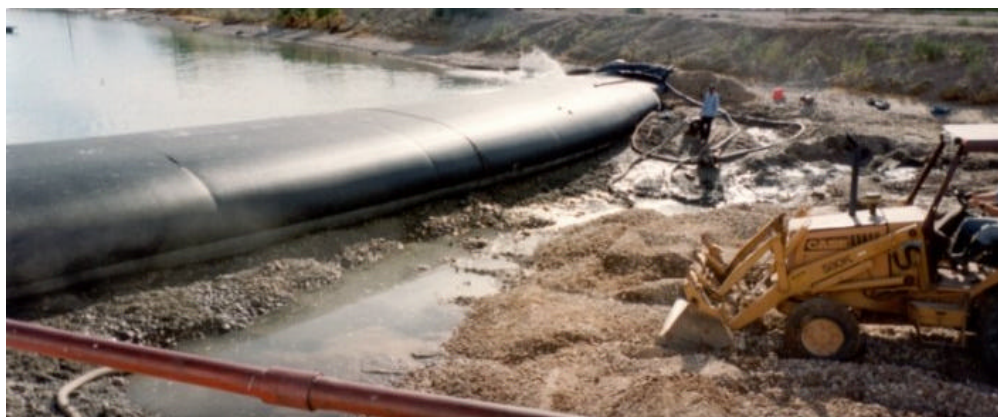
Water Structure Cofferdam - Controlling Oil with Water
