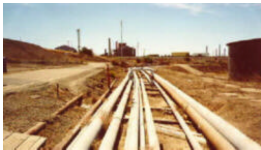
3-inch refinery inter-unit piping
