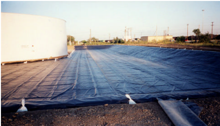
An installation of a petrogard dike liner to act as a secondary containment for industrial fluids
