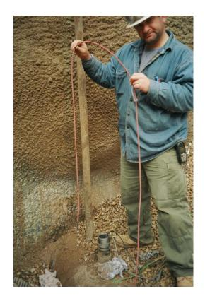
TT5000-SC or TT-FFS is inserted into end of cased road crossing
