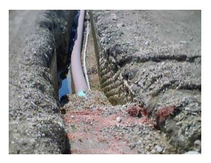
•TT5000 sensor cable is installed in slotted PVC pipe and buried beside pipeline
