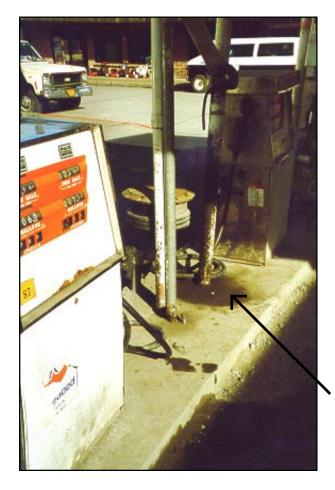
Note the "upgraded" spill bucket behind the bent pipe in center of photo. While this technically meets the requirements for spill prevention, this set up is an operational hazard. The top of the bucket cap should be flush-mounted with island surface.
