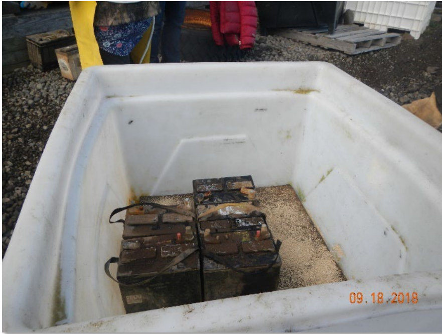
Batteries being placed in a tote with absorbent material.
