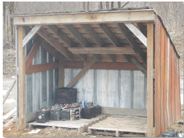
Covered storage shed for lead acid batteries.
