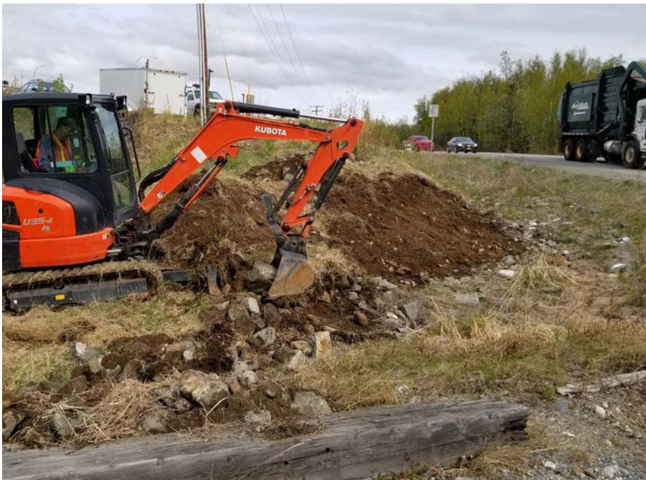
Trees were removed from under the utility lines. Riprap and stones were collected by volunteers and as part of excavation for reuse during construction of bio-infiltration cells and protecting channels from erosion.
