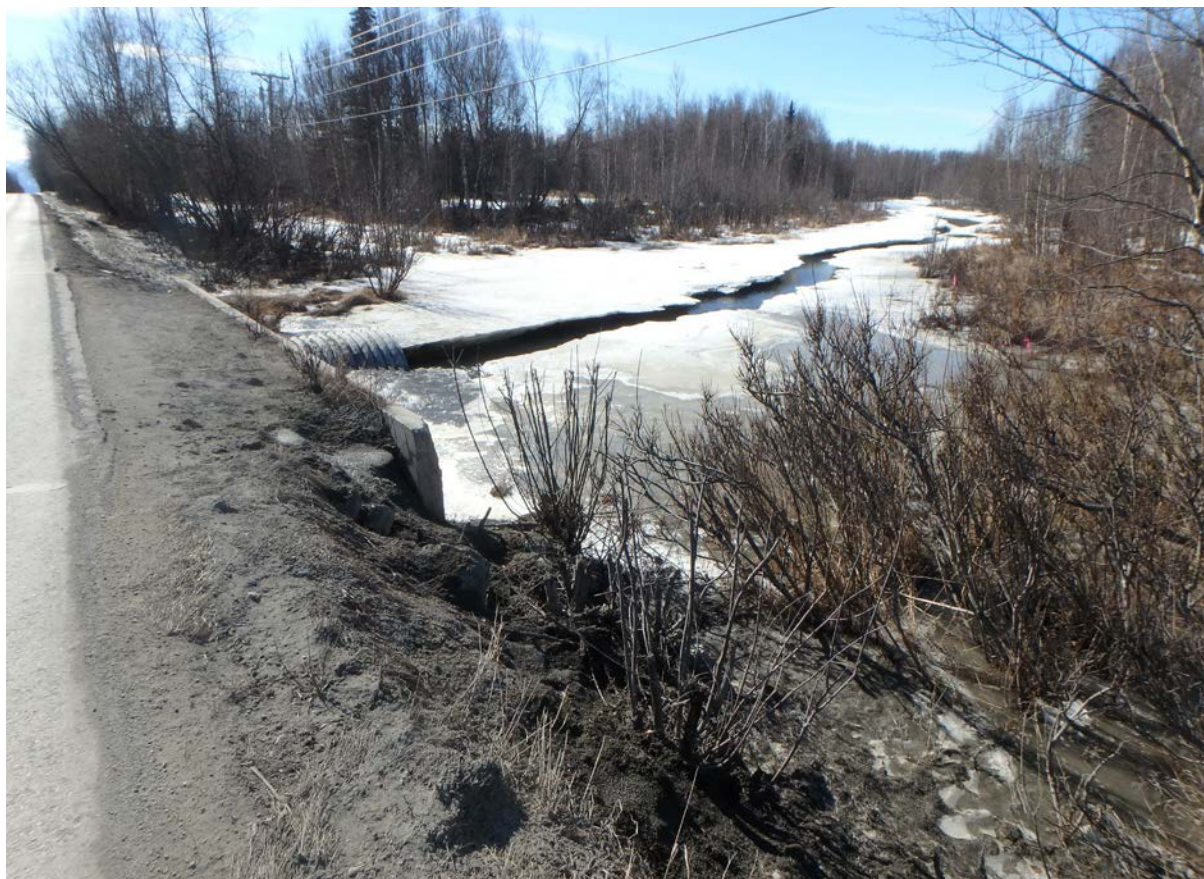
2018: Water collection in spring runoff adjacent to Fern Street contains sediment and pollutants from Knik Goose Bay Road, Palmer-Wasilla Highway, and Fern Street. The sediment and pollutants smothered native vegetation and created a sediment plume within Cottonwood Creek.
