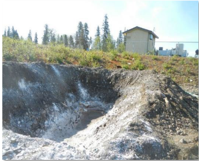
Septage trench with lime added.
