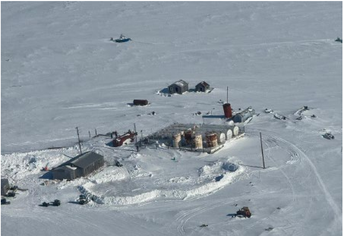
Figure 1. Overflight of spill site boundary on March 10, 2024. Photo by Resolve Marine.
