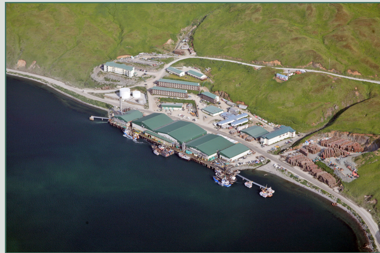
Westward Seafoods looking southeast.
