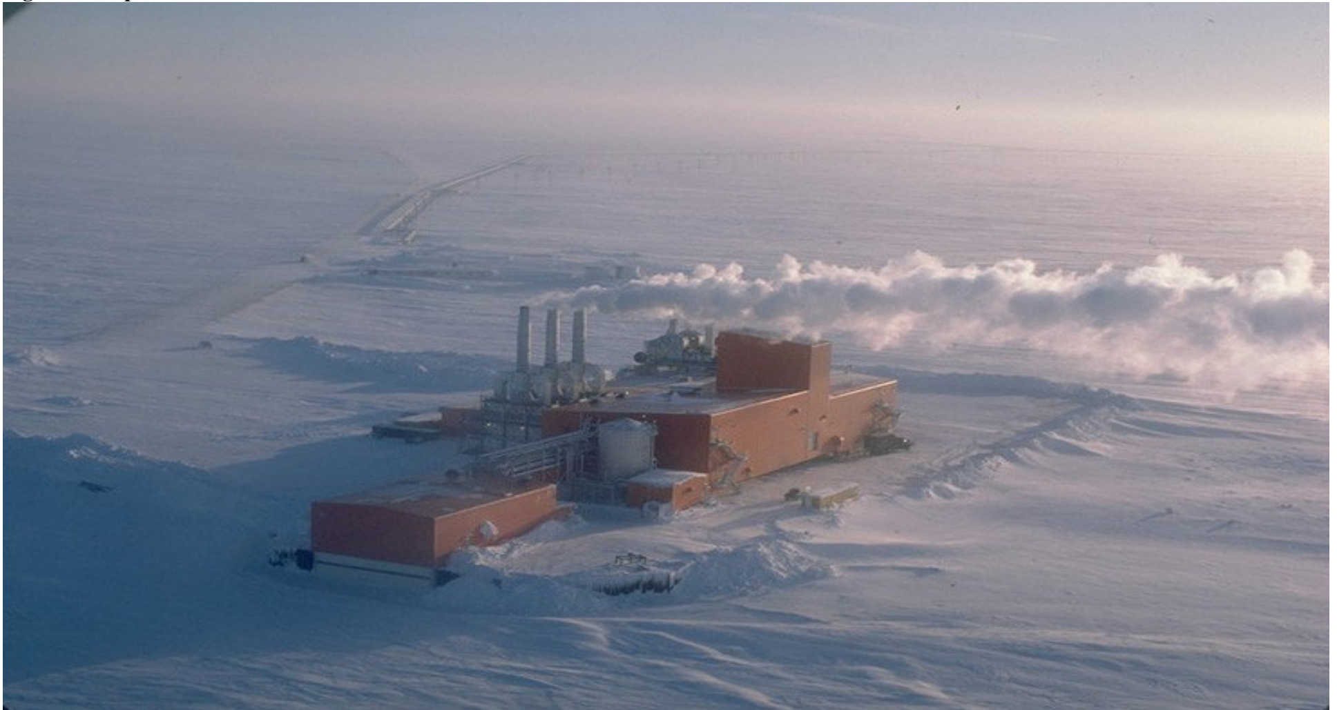
Figure 3: Kuparuk Seawater Treatment Plant
