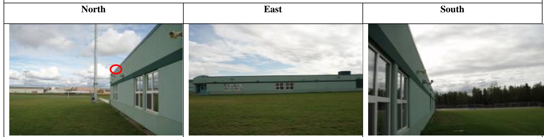
Views in three directions towards the Hunter Elementary School Site
