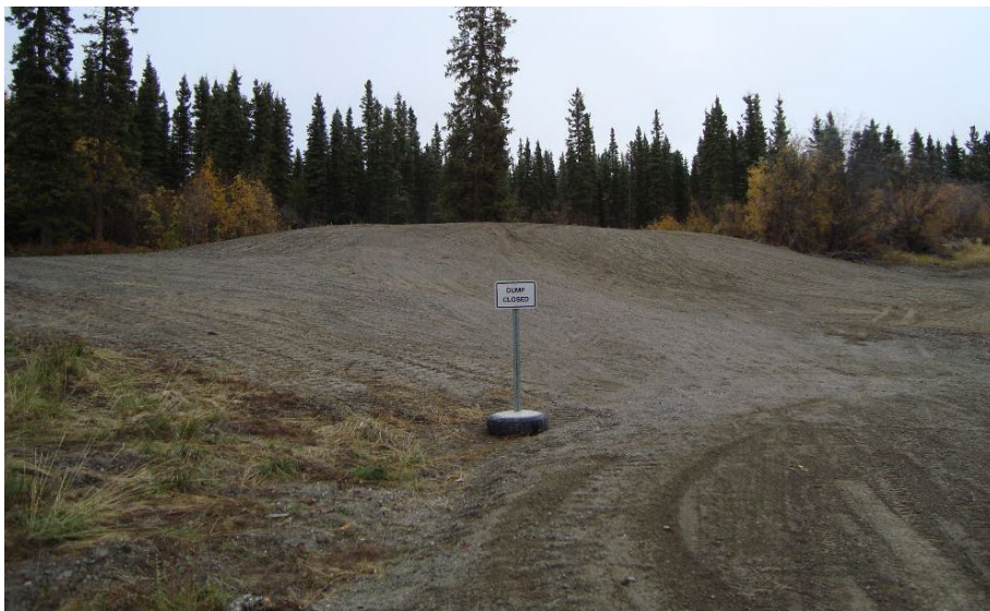
Polluted soil used to help close out a section of the landfill.
