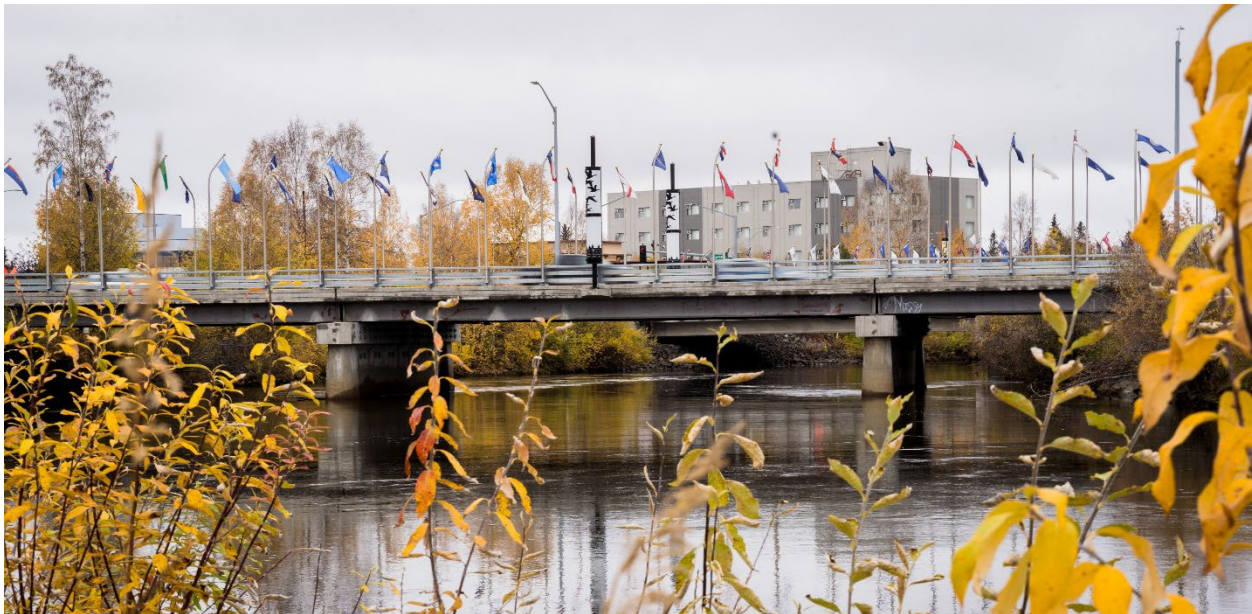
Cars drive over the Cushman Street bridge over the Chena River in downtown Fairbanks. Photo by DEC staff Jeff Fisher
