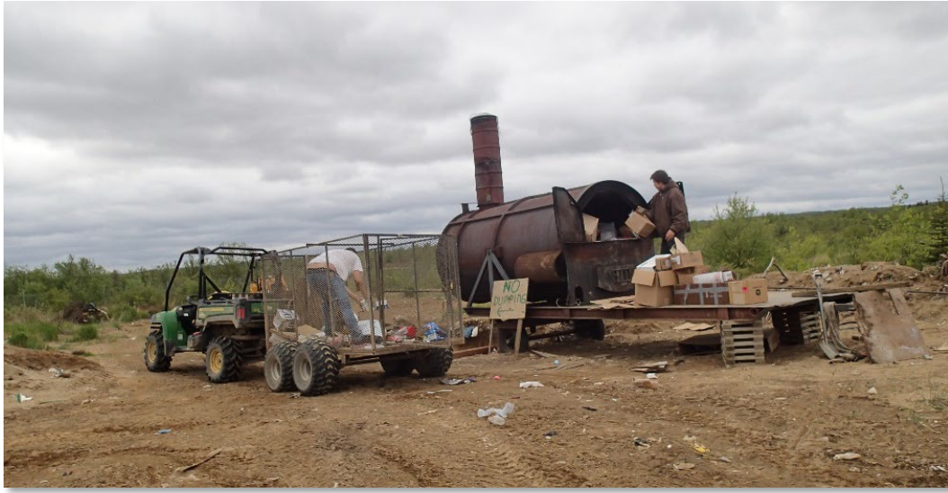
Waste transfer from the collection trailer to the burn unit by the operator.
