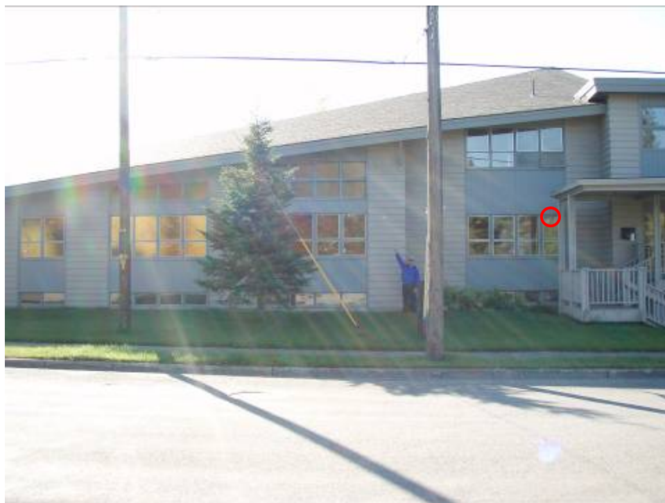
Figure 3.2:3: View of CO probe at Garden Site. The red circle indicates where the probe is located.
