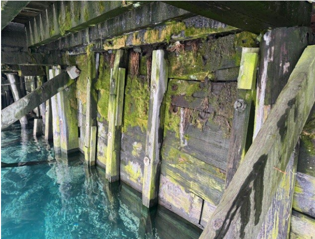
Existing wood bulkhead
