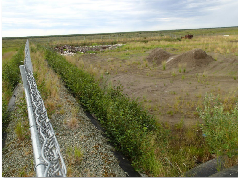
Above-grade area fill surrounded by wetlands.
