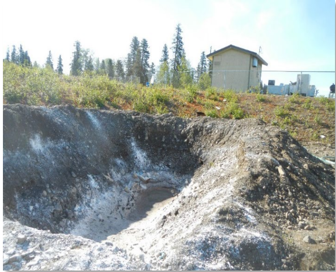
Septage trench with lime added.
