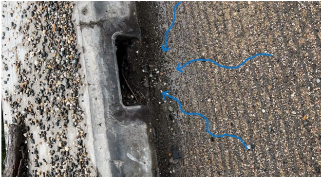
OPEN SCUPPER (ON BRIDGE DECK)
