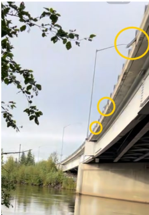
Scupper outfall on Riverside
