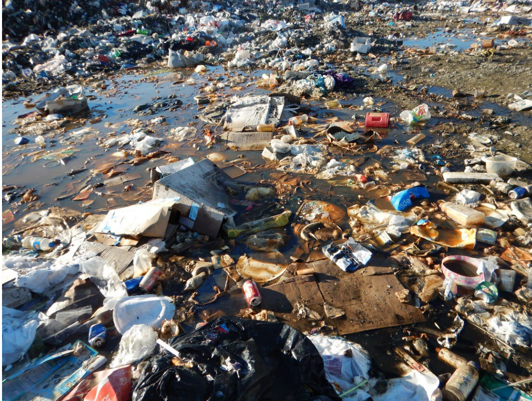
Leachate, as indicated by red and orange staining, where the waste and water are in contact.
