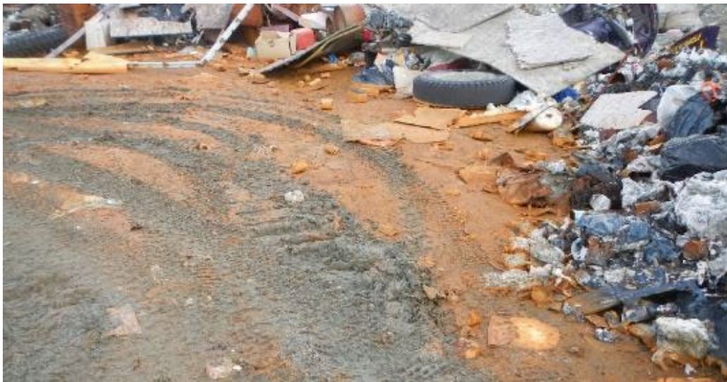
Orange staining near the waste caused by leachate. The waste should be covered to prevent the formation of leachate.
