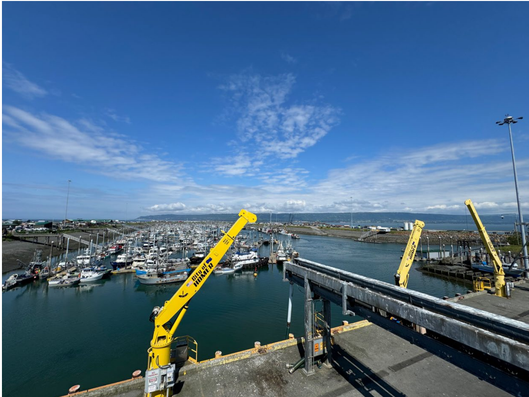
Figure 14: Homer harbor seen from above. Cranes in the foreground are available to the public for vessel operations.
