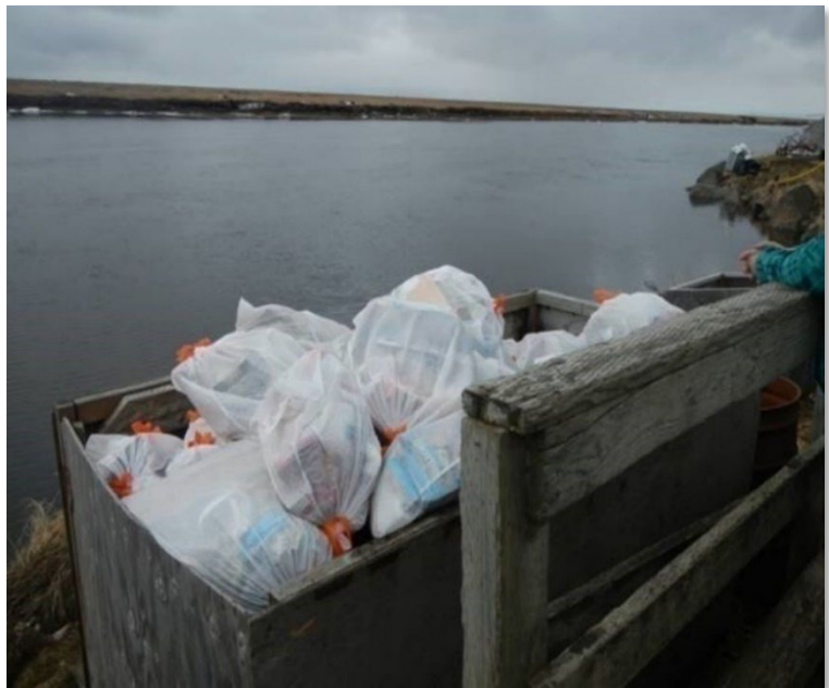
Waste collection bins for a landfill on the river. These bins are emptied by the operator in the winter preventing the buildup of waste on the riverbank from residents disposing of waste from their boats. These bins should be covered to prevent litter and water infiltration.
