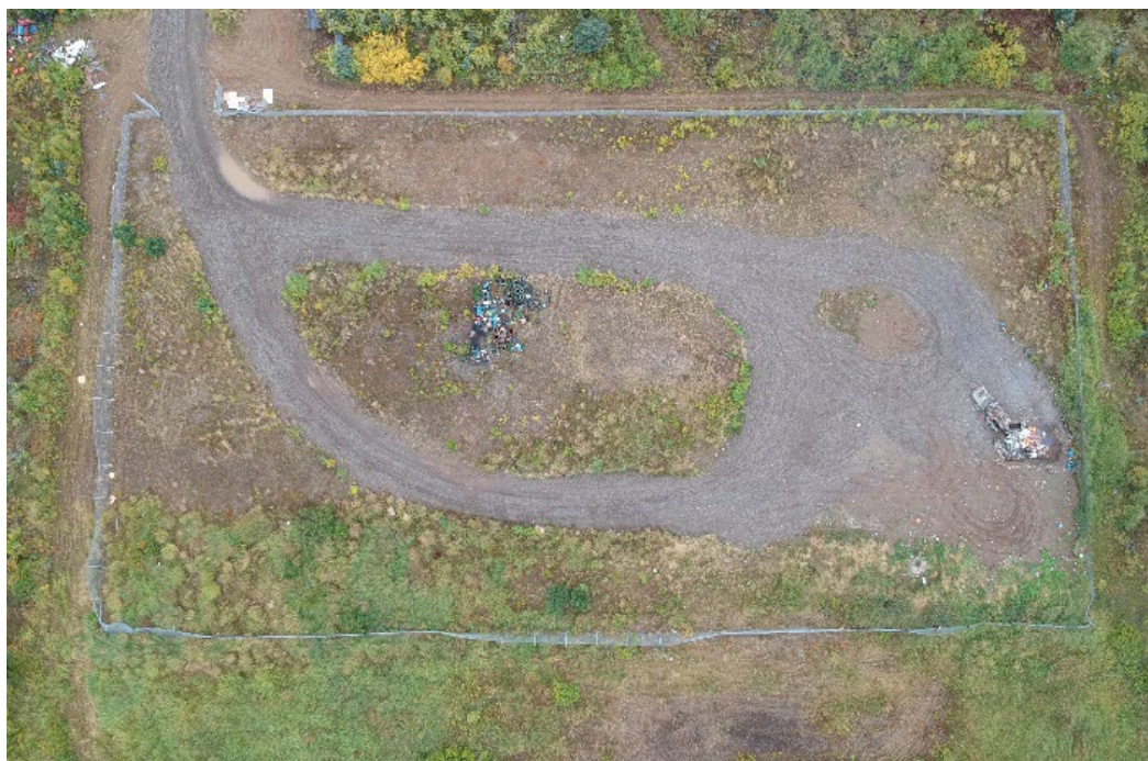
Well-maintained road within the landfill.
