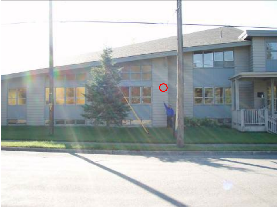
Figure 2.2:3: View of CO probe at Garden Site. The red circle indicates where the probe is located.
