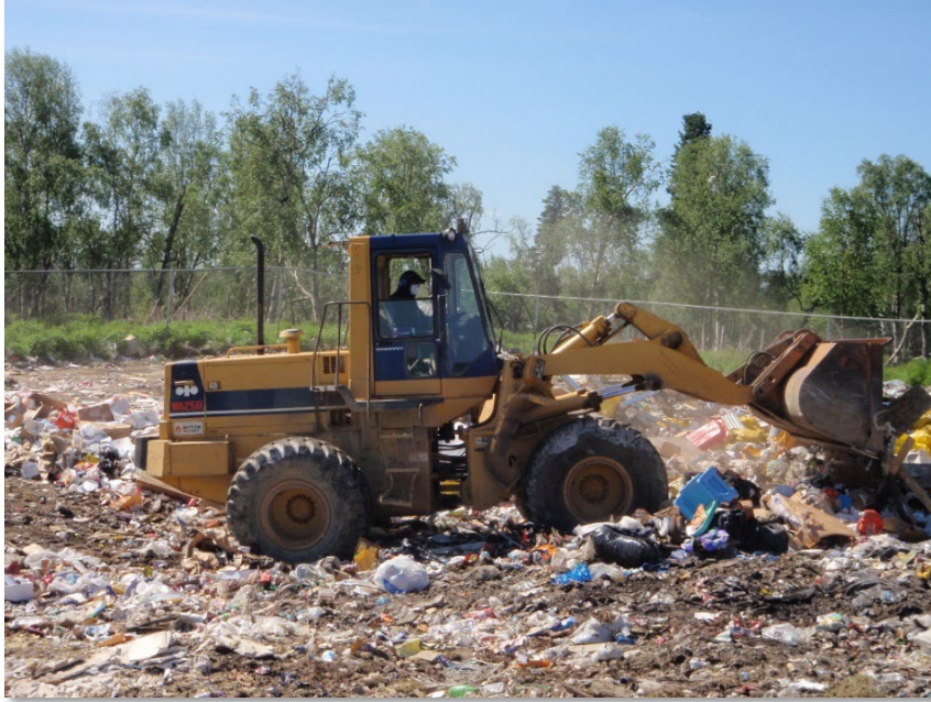
Landfill operator consolidating waste.
