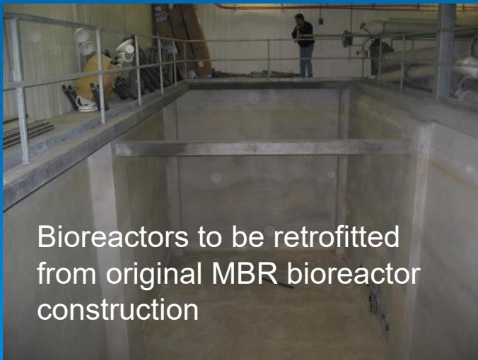
Bioreactors to be retrofitted from original MBR bioreactor construction
