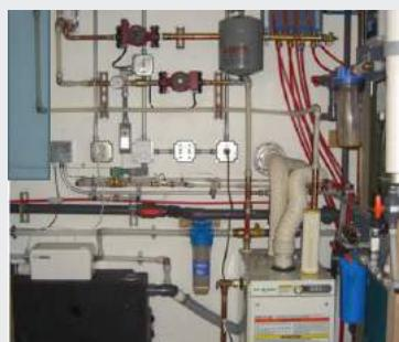
Waste water storage tank, drinking water filters and freeze-thaw protection using heat trace pipes
