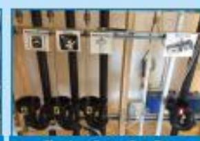
Plumbing Fixture Drop Pipes
