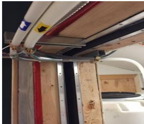
Accordion-Type Flexible Joint
