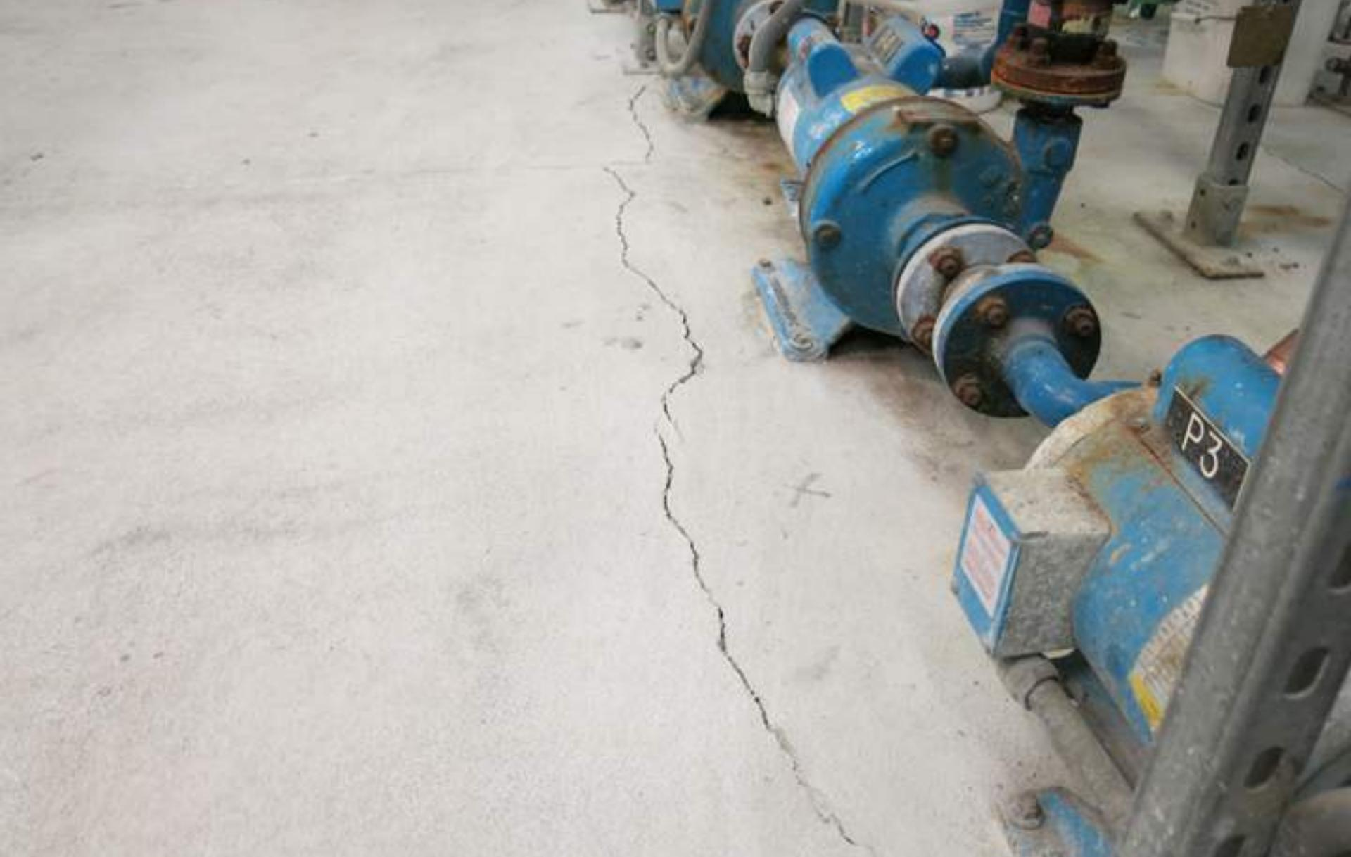
In Noatak, failing foundations from permafrost warming
