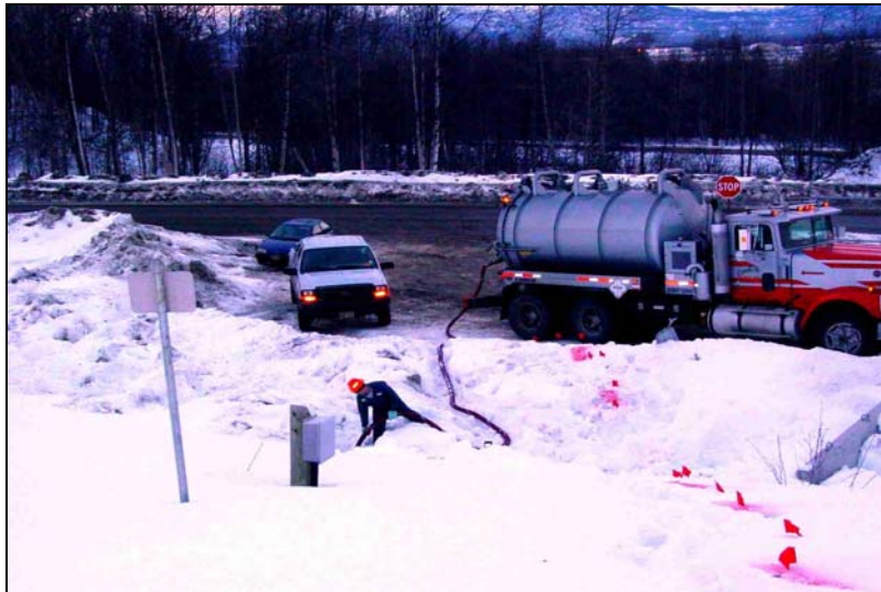
EAFB Fuel Recovery of Jet Fuel with vacuum truck.
