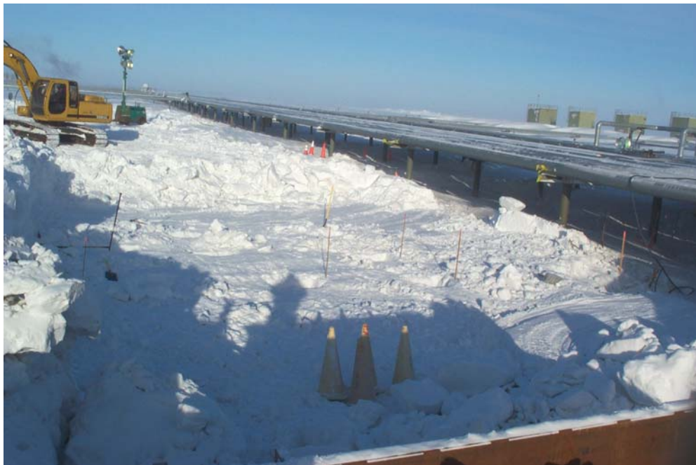
Figure One – Photo taken by BPXA of the spill site.
