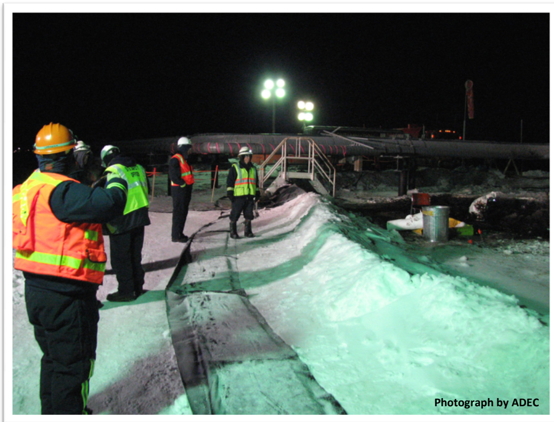
Work crew working around location being steam treated, December 7, 2009.
