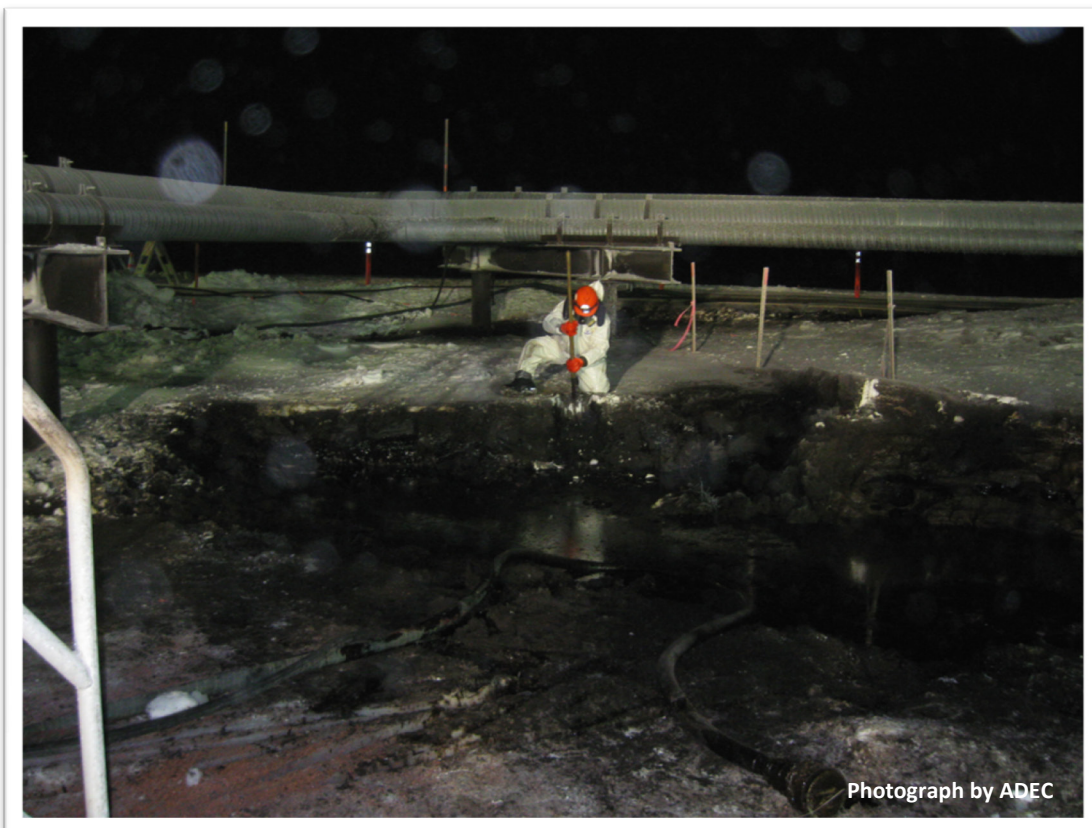
Work crew working around location being steam treated, December 7, 2009.
