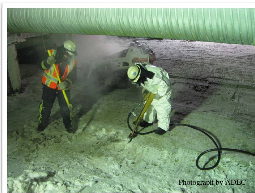
Workers use jackhammers under the pipeline to remove contaminated ice.
