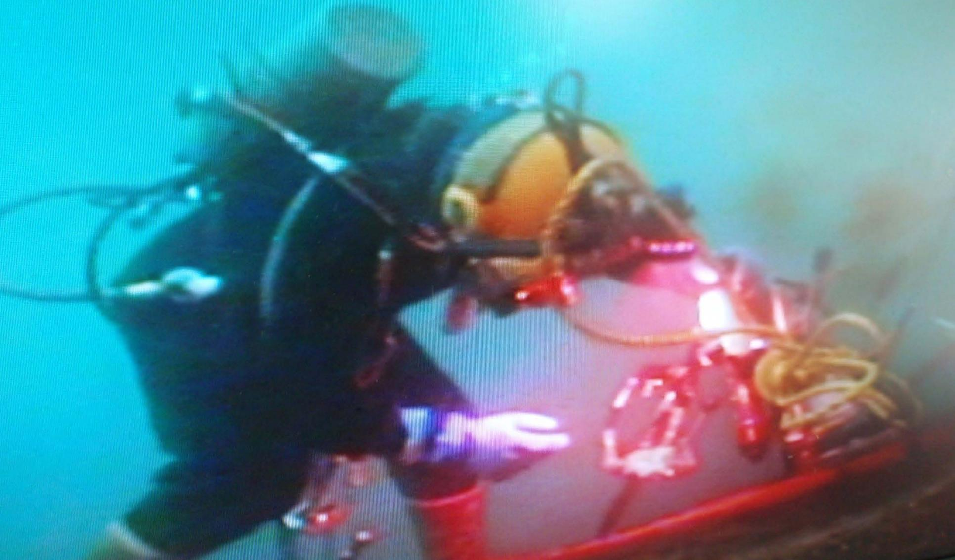
Since oil floats, the first hole is drilled near the top of the tank. If oil is present in the first hole, they know there is some amount of oil in the tank.
